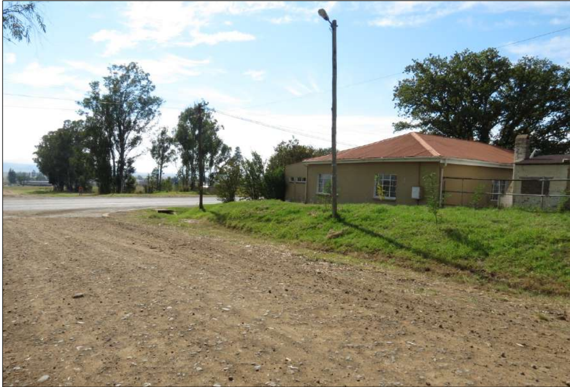
Figure 31 – General view of the old dwelling at Mat 8. The road reserve ends immediately adjacent to the façade of the building visible in this photograph.
