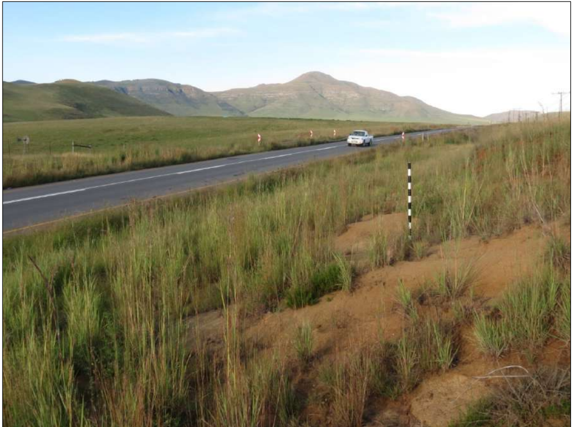
Figure 27 – General view of Mat 6.
