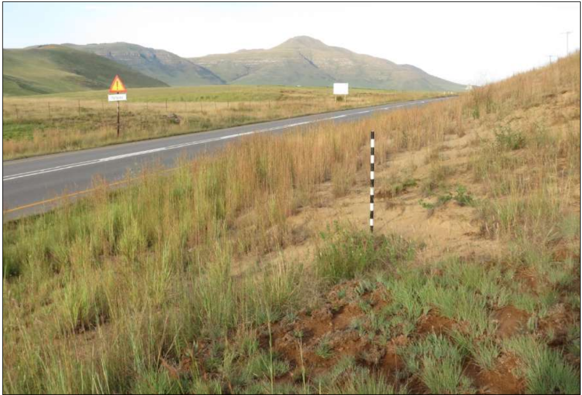
Figure 29 – General view of Mat 7.
