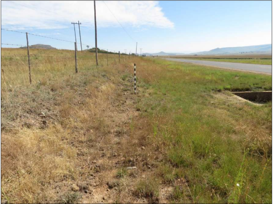
Figure 35 – General view of MAT 10.
