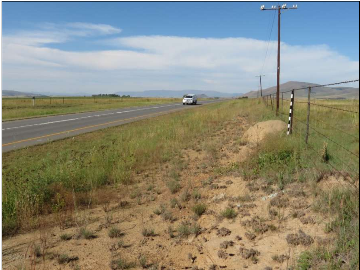
Figure 23 – General view of Mat 4.
