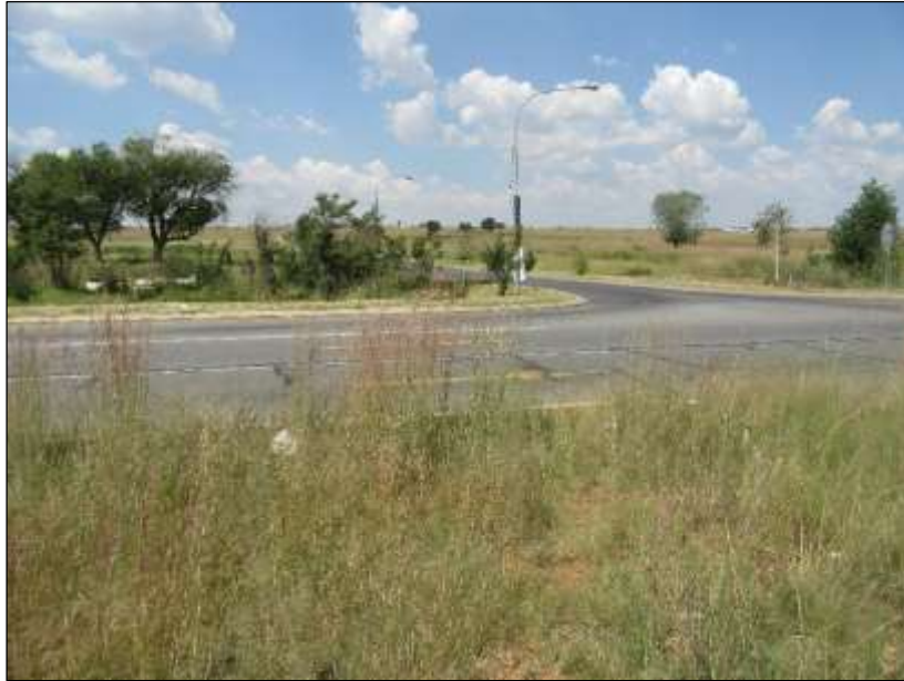
Figure 3: Figure 2: Close view east of the junction of the Heidelberg Rd (in the background) and Shakwane St (Alternative Site 1).
