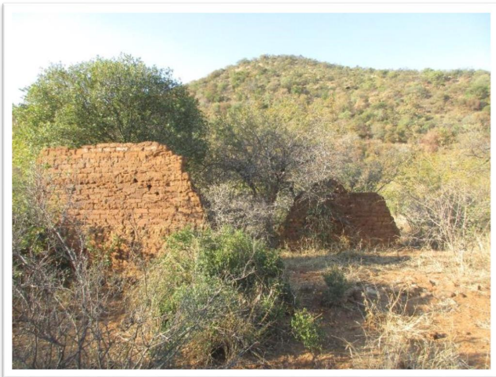
Figure 16 : The wall remains of the old Lutheran Church (Site S4).
