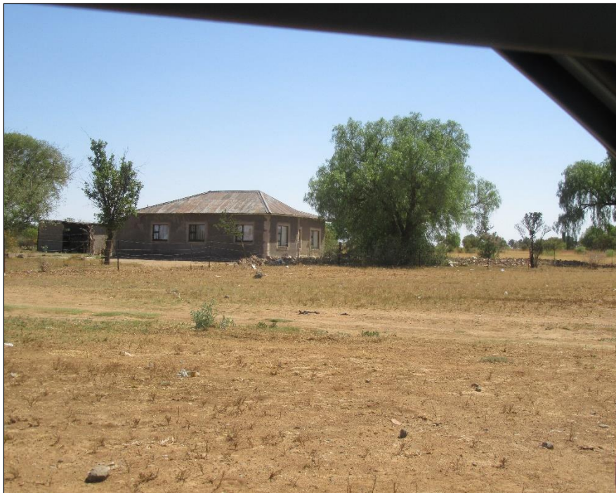
Figure 9: Residential building with pitched roof of corrugated iron sheets.
