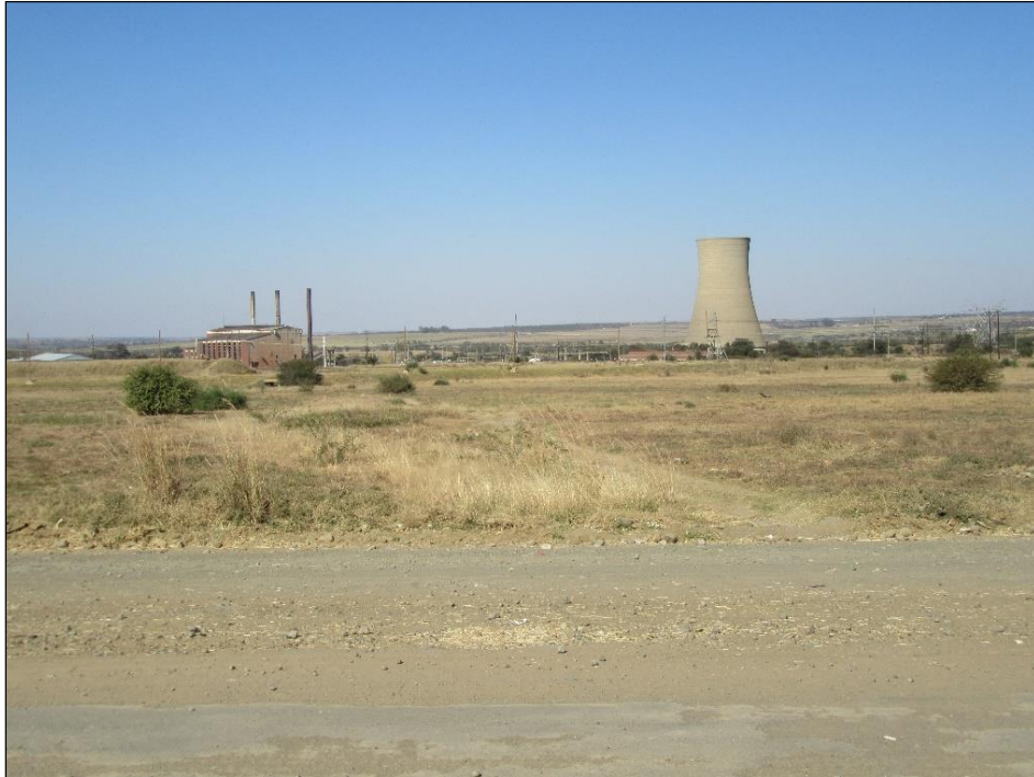
Figure 8: The Old Kroonstad Power Station is a historical landmark located in Industria east of Brent Park.
