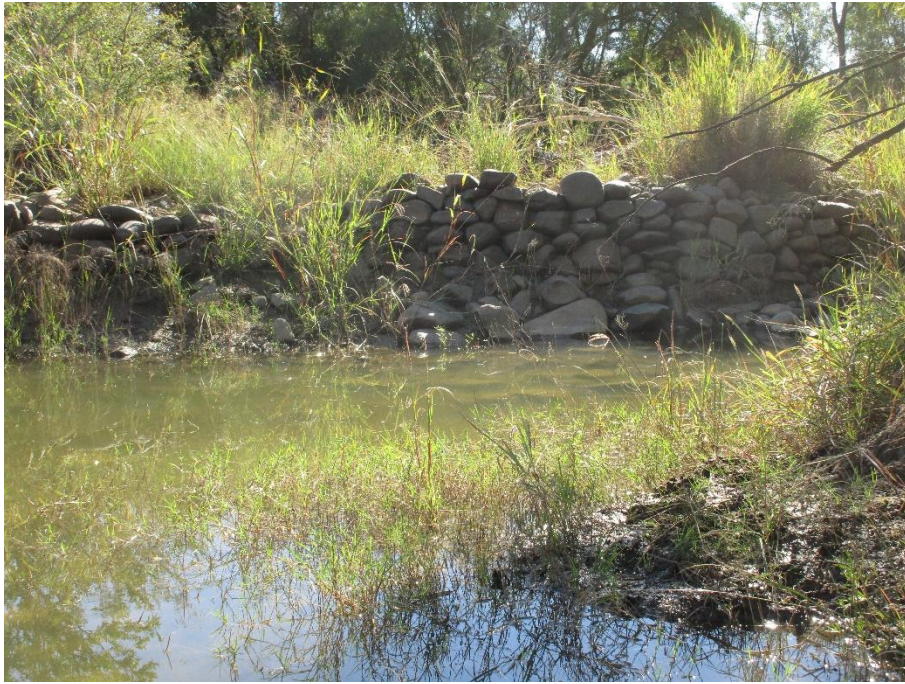
Fig 9. Platform revetment wall used for mining (Site 2).
