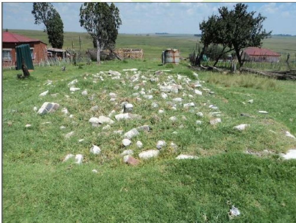
Photo 12: D02 Foundation Remains
