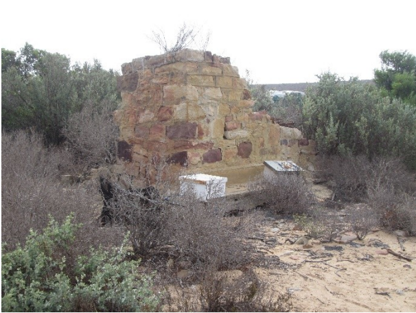
Figure 37: View Towards the northwest of the third ruin, presumably an outbuilding, at De Boom 2018/002 (waypoint 002).
