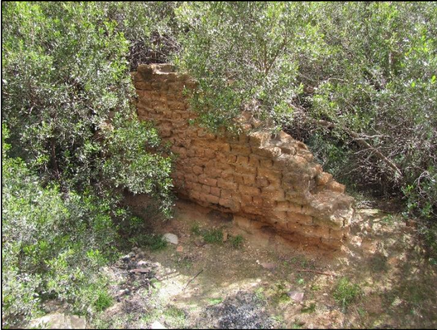
Figure 18: Ruined structure at waypoint 261. It has mud brick walls on a stone foundation.
