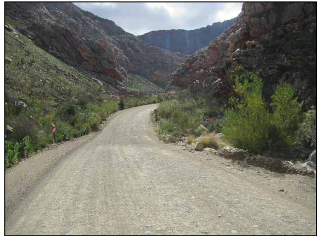
Figure 12: View towards the northeast in the northern part of the pass.
