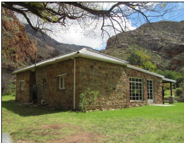
Figure 33: View of the historical stone cottage On the Aristata Farm at waypoint 260.
