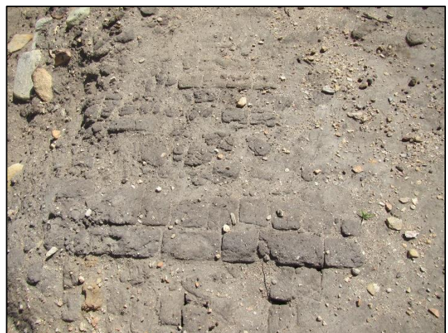
Figure 21: Detail of collapsed mud brick walling
