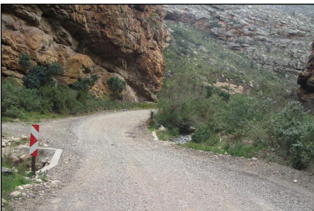
Figure 6: Current river crossing at km 50.8.
