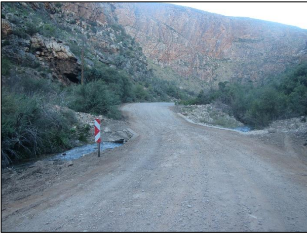
Figure 4: Current river crossing at km 53.4. Note small culvert and exposure of road to river.
