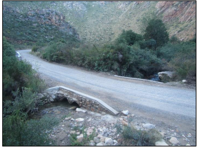
Figure 3: Current river crossing at km 54.1. Note small pipes for river.
