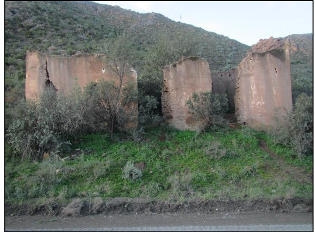
Figure 19: Ruined structure at waypoint 219. It is built of mud bricks.
