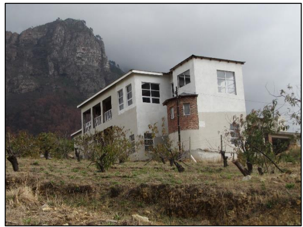
Figure 21: The house just north of the site.
