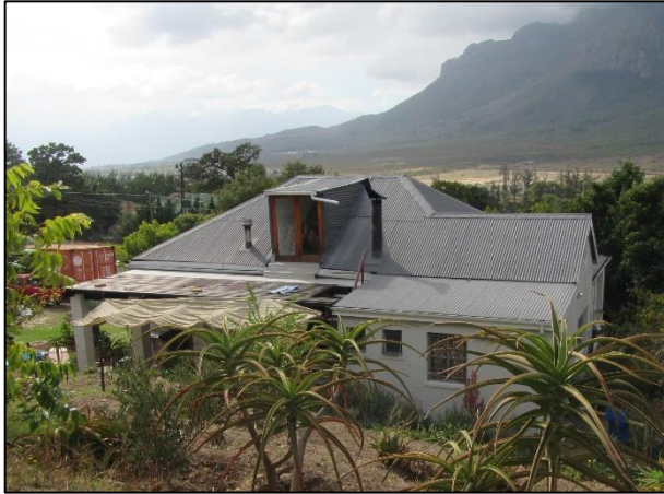
Figure 18: View of the dwelling on Farm 1202/1 as seen from behind (facing east).
