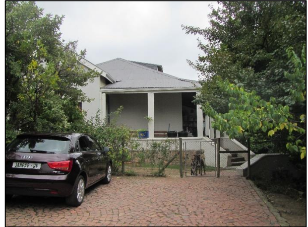
Figure 19: View of the dwelling on Farm 1202/1 from the side (facing north).
