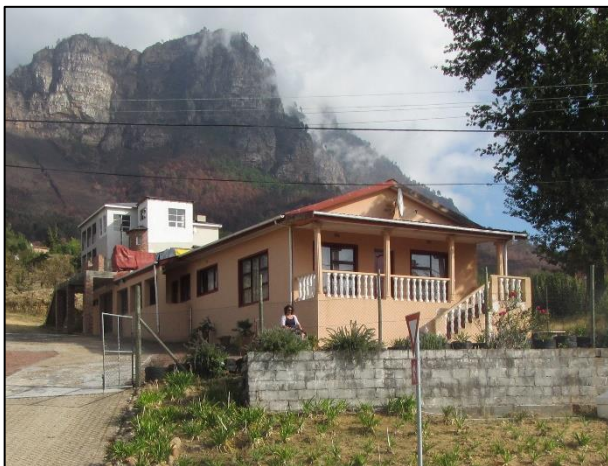
Figure 20: The house immediately adjacent to the site on Helshoogte Road.
