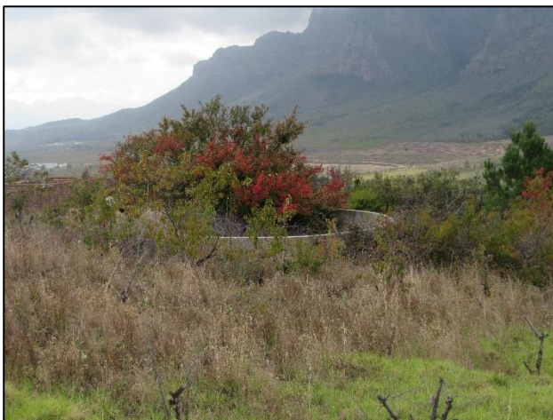
Figure 12: Cement reservoir on the site.
