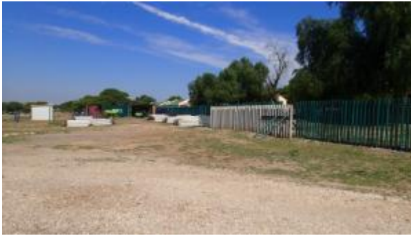
Photograph 1: Component 1 - Concrete Pole Fence around Core Area under construction.
