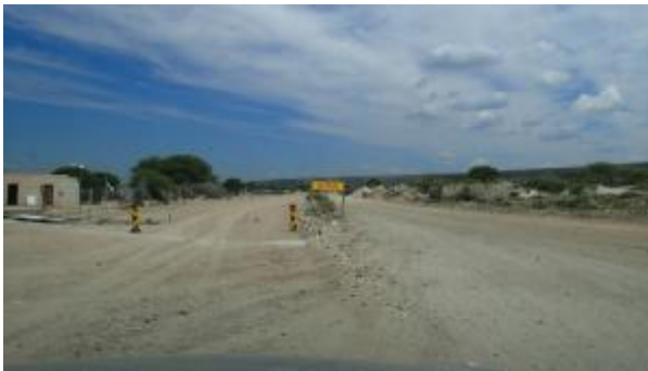
Photograph 5: Component 4 - Road to Thomeng is under construction.
