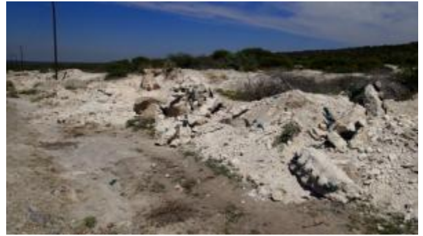
Photograph 2: Component 1 - Previous fence needs to be disposed of appropriately.
