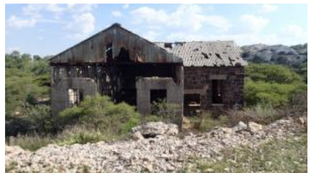
Photograph 8: Component 7 - Power House to be restored.
