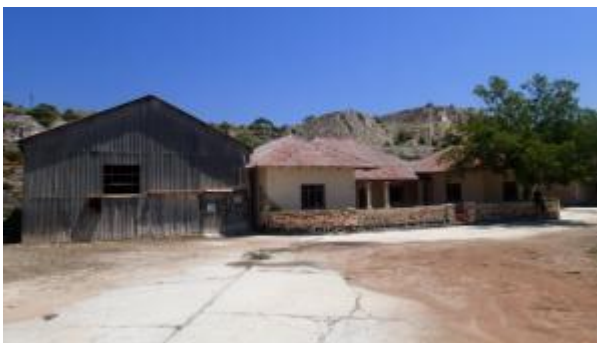
Photograph 7: Component 6 - Mine Manager's Office to be restored.
