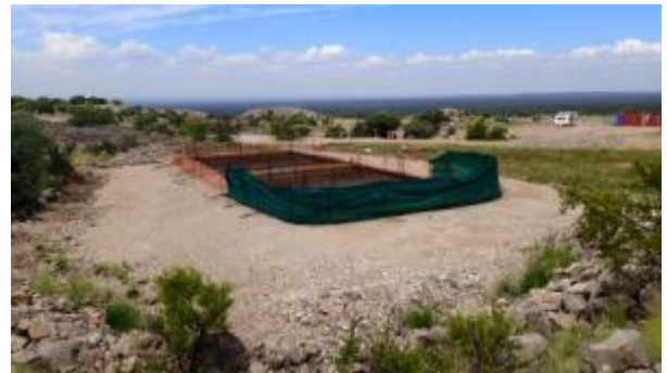
Photograph 4: Component 3 - The ablation facility at Thomeng Falls is under construction.
