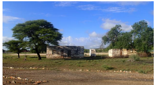
Photograph 4: Stone building at current Entrance.
