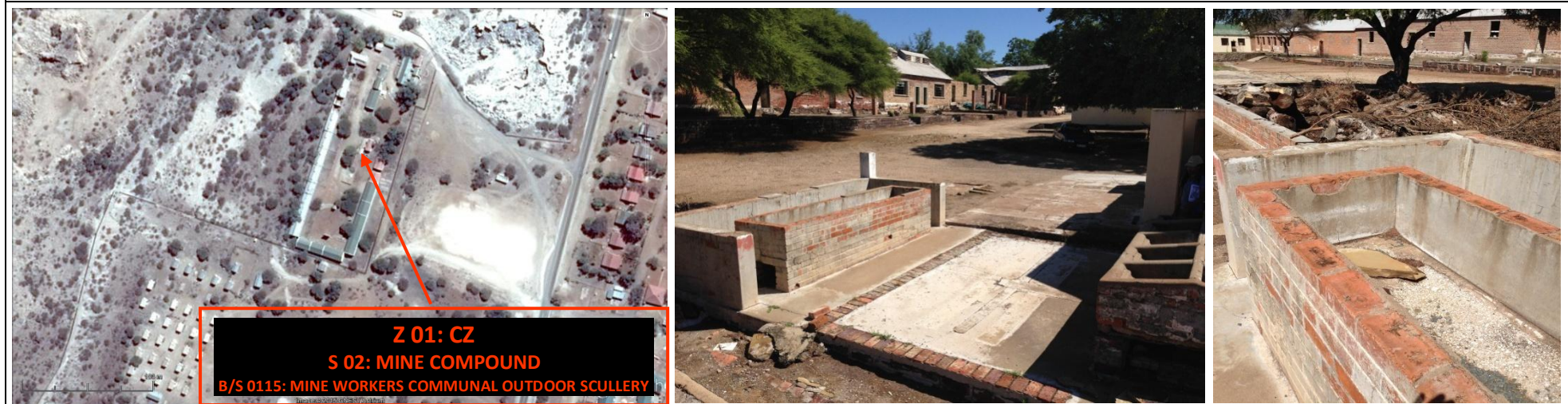
FIGURE 15 • PHOTOGRAPH 15 • Zone 01 [Z 01]: Core Zone [CZ] • Site 02 [S 02]: Mine Compound Complex • Building/Structure 0115 [B/S 0115]: Mine Workers Communal Outdoor Scullery • Date: 24 February 2015
