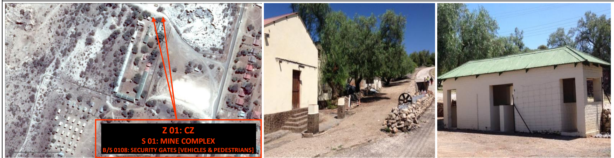
FIGURE 08 • PHOTOGRAPH 08 • Zone 01 [Z 01]: Core Zone [CZ] • Site 01 [S 01]: Mine Compound Complex • Building/Structure 0108 [B/S 0108]: Security Gates [Vehicles & Pedestrians] • Date: 24 February 2015
