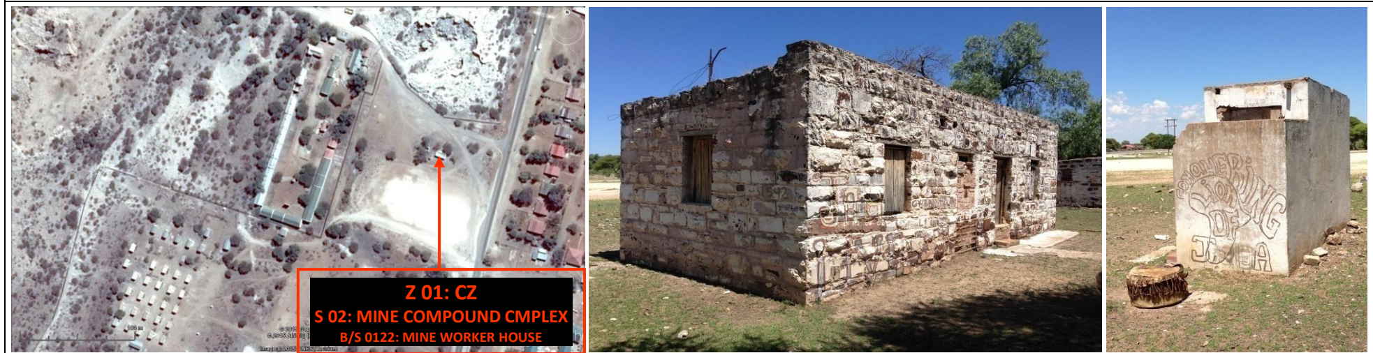
FIGURE 22 • PHOTOGRAPH 22 • Zone 01 [Z 01]: Core Zone [CZ] • Site 02 [S 02]: Mine Compound Complex • Building/Structure 0122 [B/S 0122]: Mine Worker House • Date: 24 February 2015
