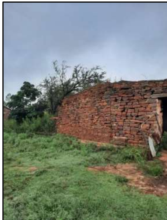
Figure 8.5. Kraal structure in the farmstead complex.
