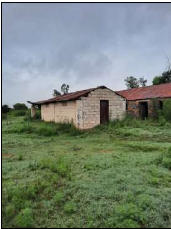
Figure 8.4 Recent additions at the farmstead complex DH 002.
