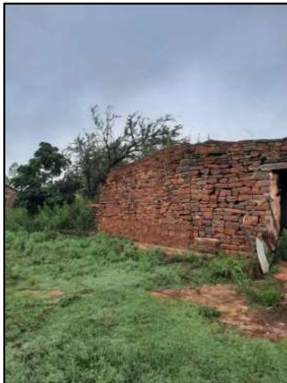
Figure 8.5. Kraal structure in the farmstead complex.
