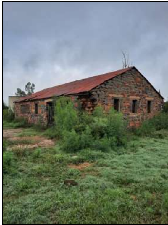
Figure 8.3. Main house – alternative view.
