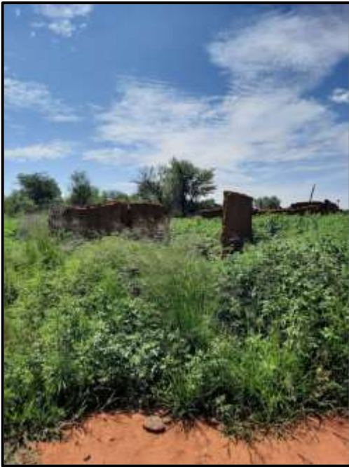
Figure 8.6. Degraded mudbrick structure at R003
