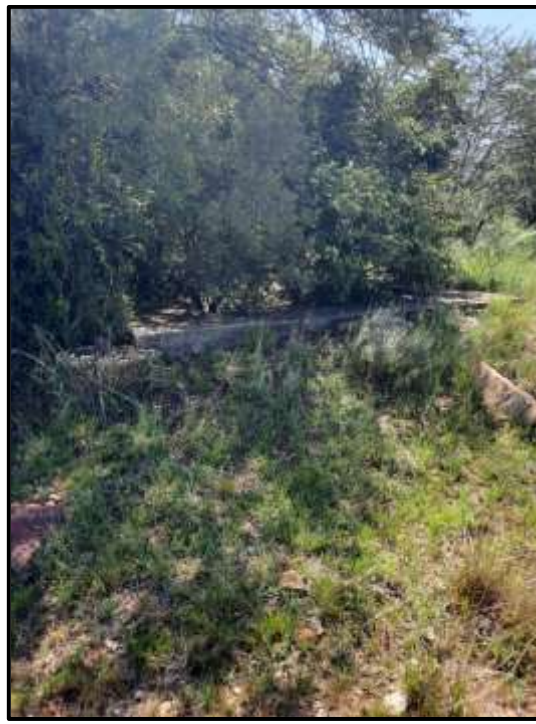
Figure 8.9. Shaft entrance at R007.
