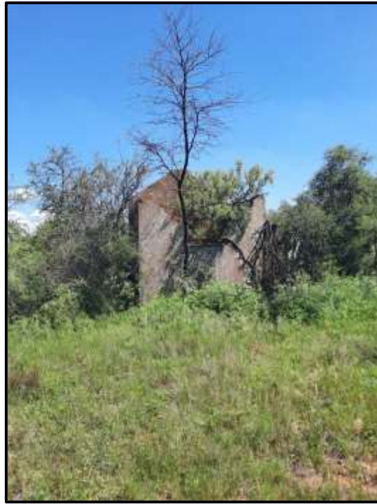
Figure 8.7. Various degraded structures occur at R007.
