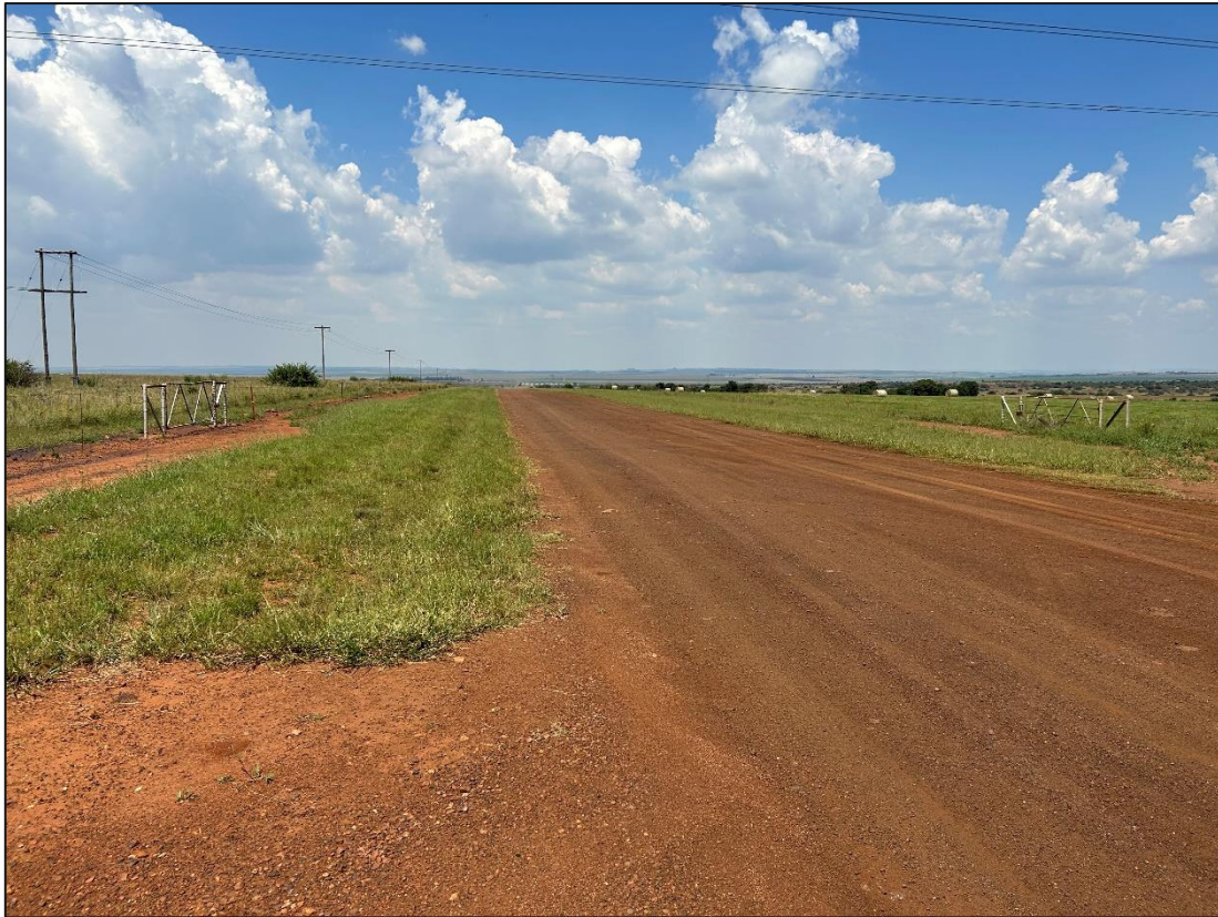
Figure 4.13: Gravel road providing access to site, taken towards the east
