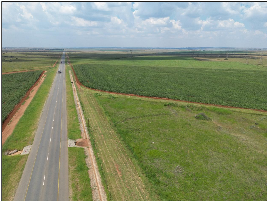
Figure 4.12: N14 national road close to site, taken towards the east
