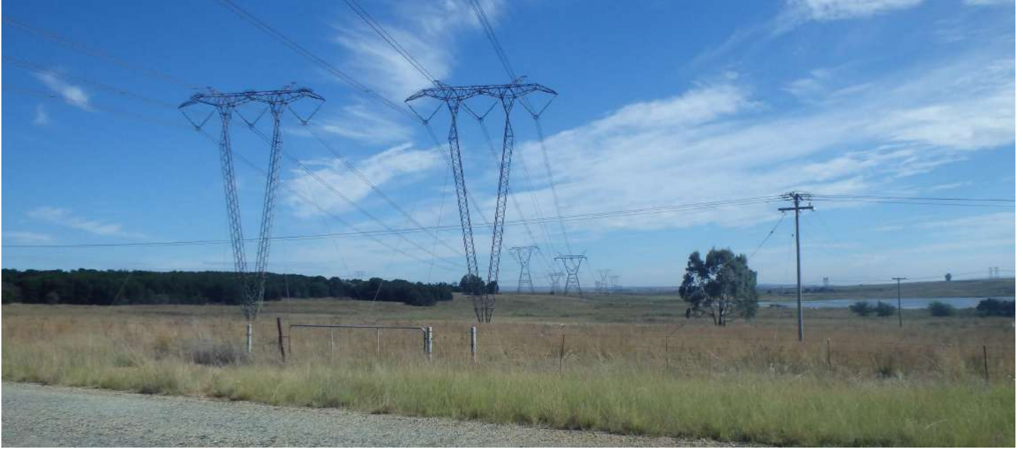
Figure 4.2: view of the large overhead powerlines crisscrossing the study area that connect to Pluto substation
