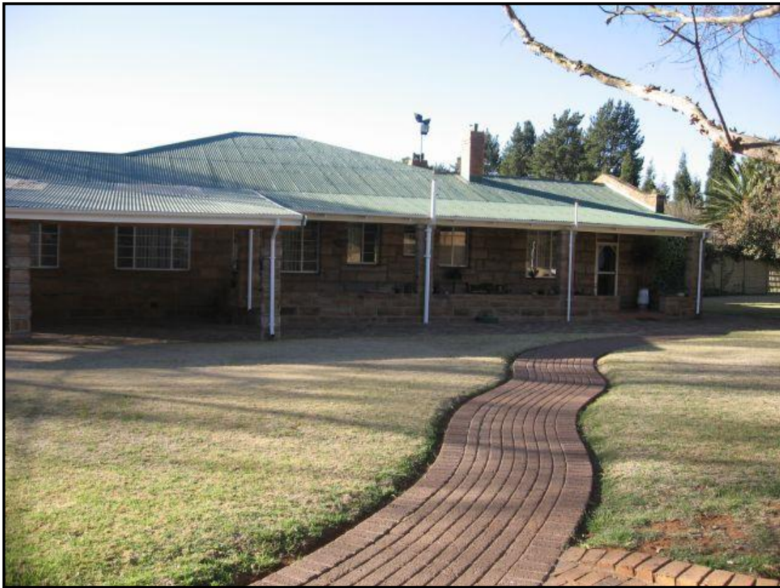
Figure 27 - View of main house
