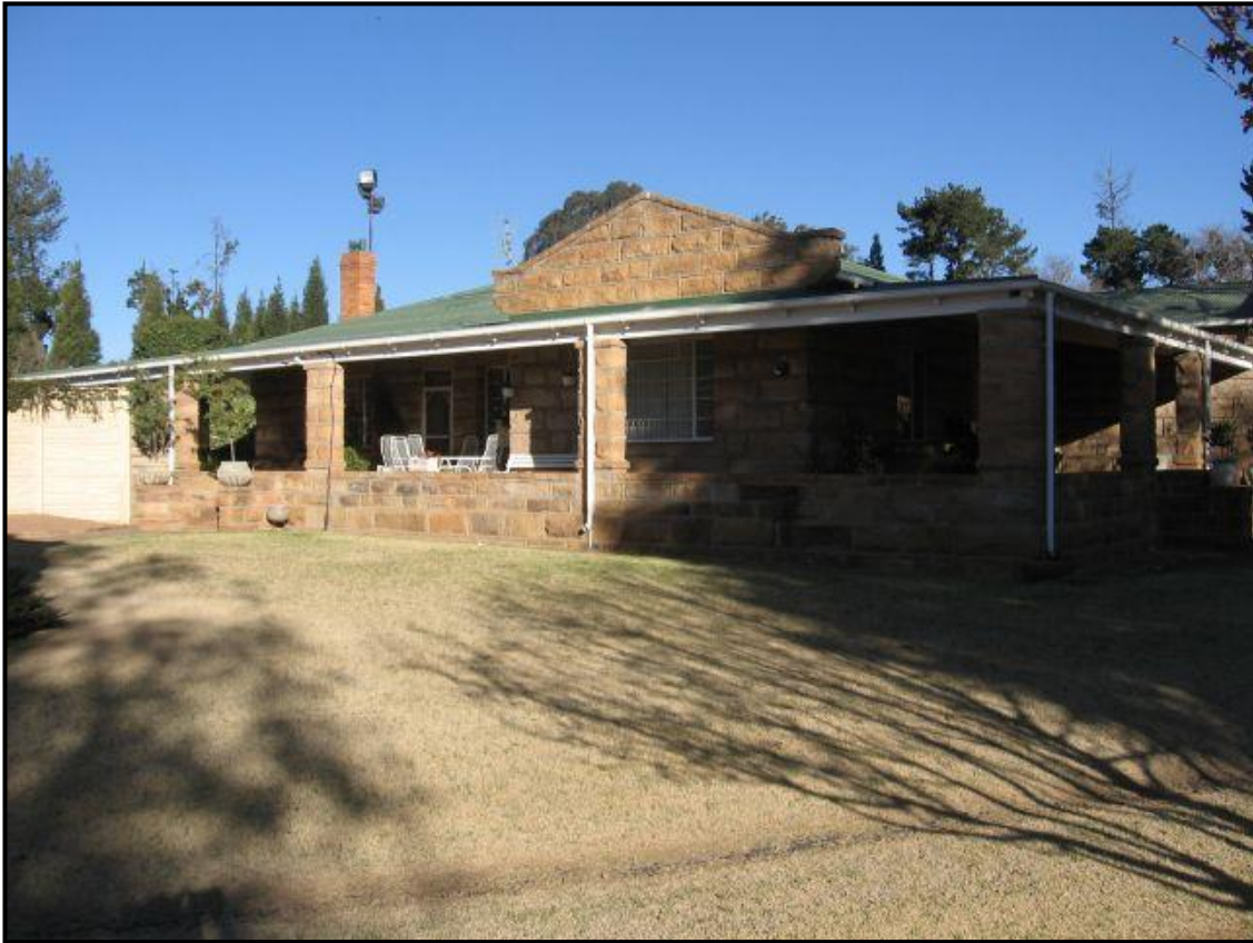
Figure 28 - View of main house from side angle
