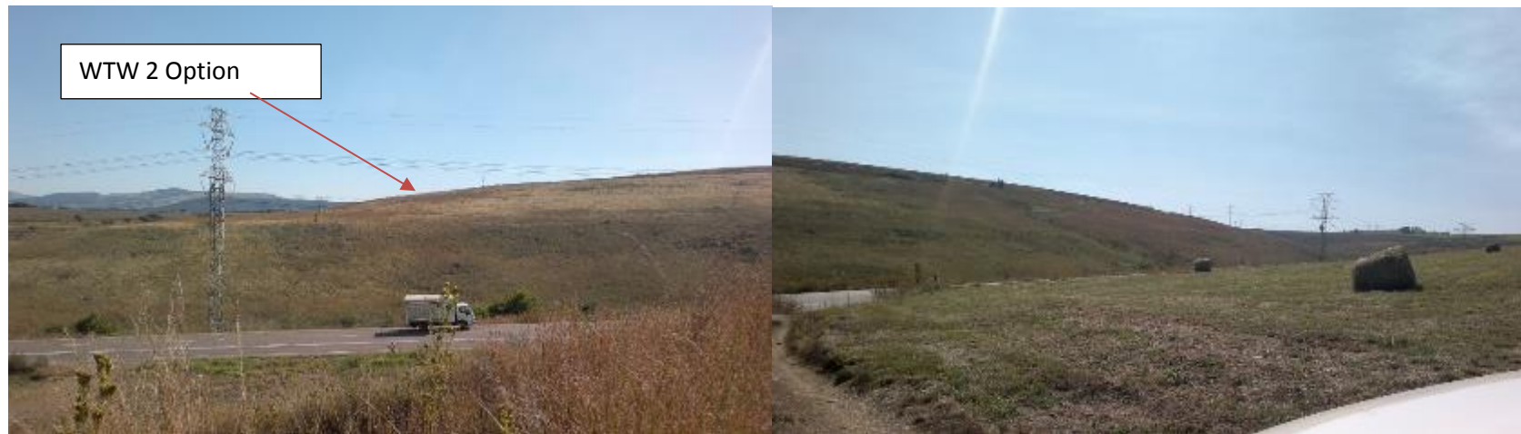
Figure 5: Panoramic view of WTW Option 2 with R56 road in foreground
