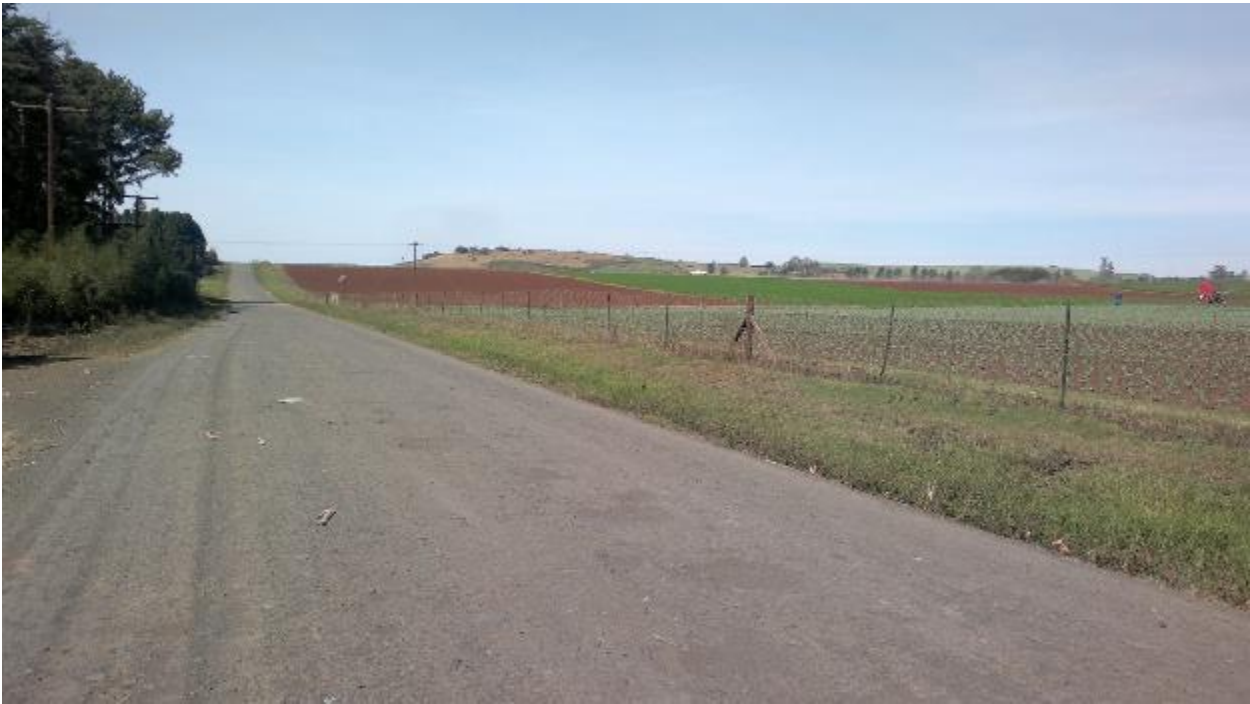
Figure 12: Section of Route Option 1 next to D360 road looking in a south easterly direction
