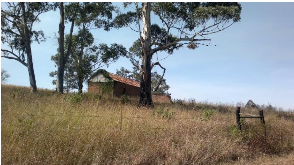
Figure 23: Structure situated south-west of pipeline link WTW2
