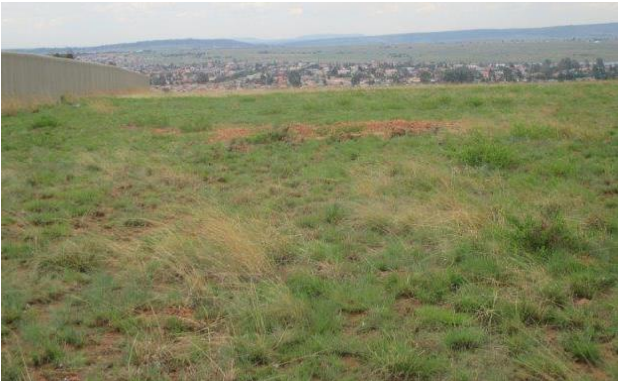
Figure 3: North western boundary fence of existing reservoir and test pit excavation of new site
