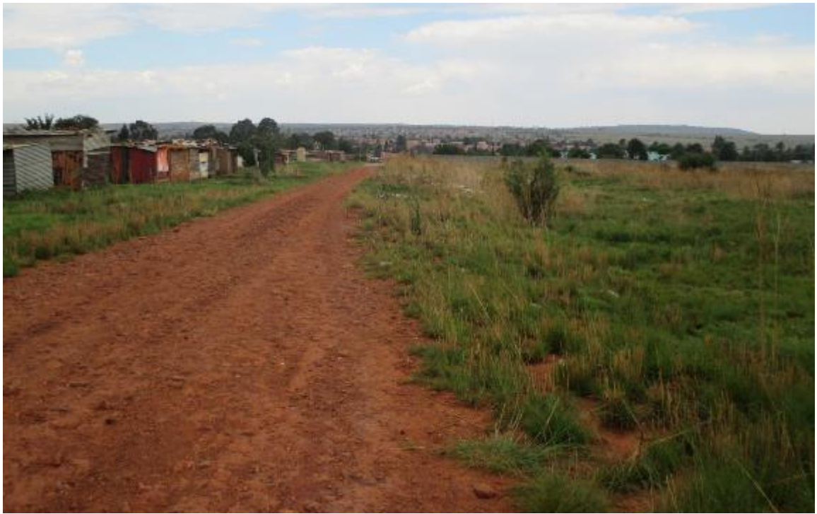
Figure 9: Scour pipeline Route 1 after Hospital Hill reservoir
