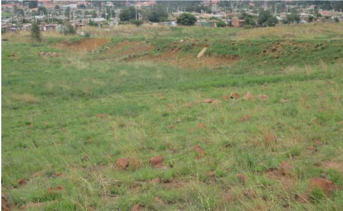
Figure 7: Old dam wall
