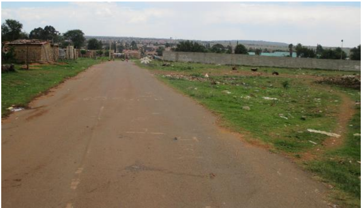
Figure 10: Scour pipeline Route 1 after Hospital Hill reservoir
