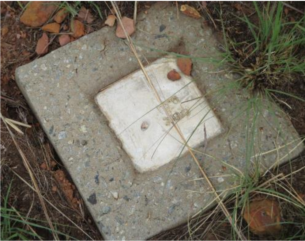
Figure 6: Concrete square indicating presence of cables
