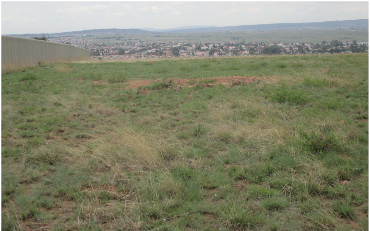
Figure 3: North western boundary fence of existing reservoir and test pit excavation of new site
