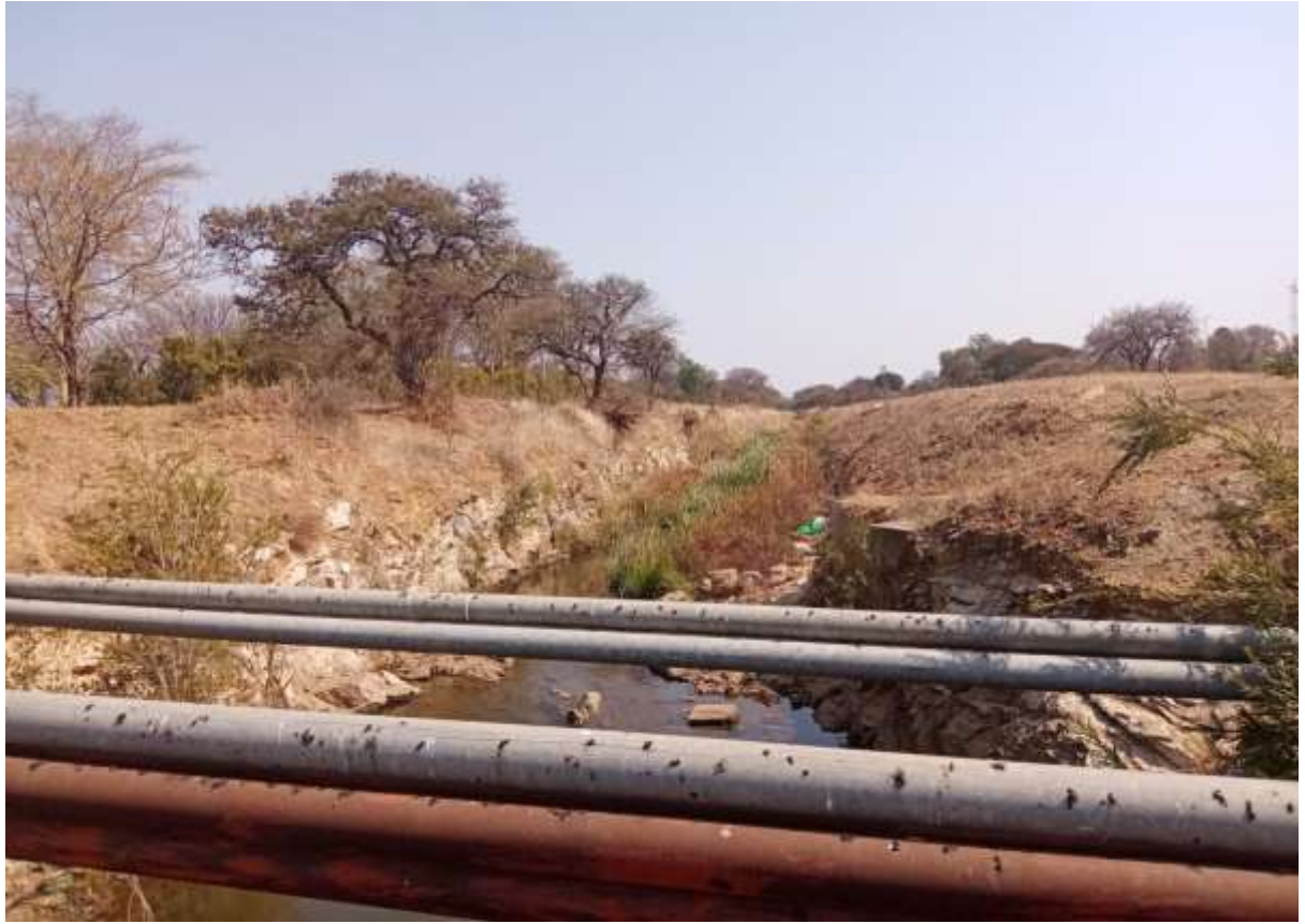
Figure 5: View of the existing municipal water channel
