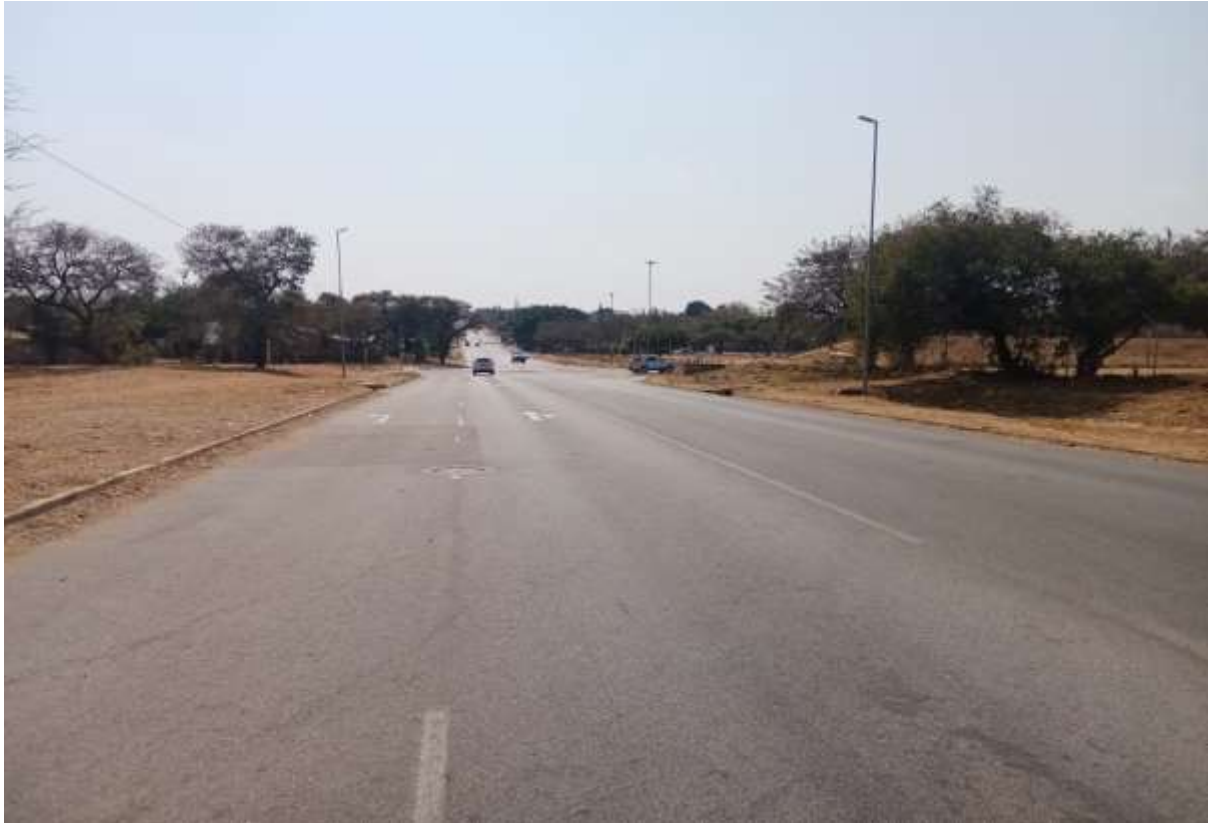
Figure 4: A southern view of Webster Street where the proposed pipeline will be laid underneath the road to connect with the existing water channel
