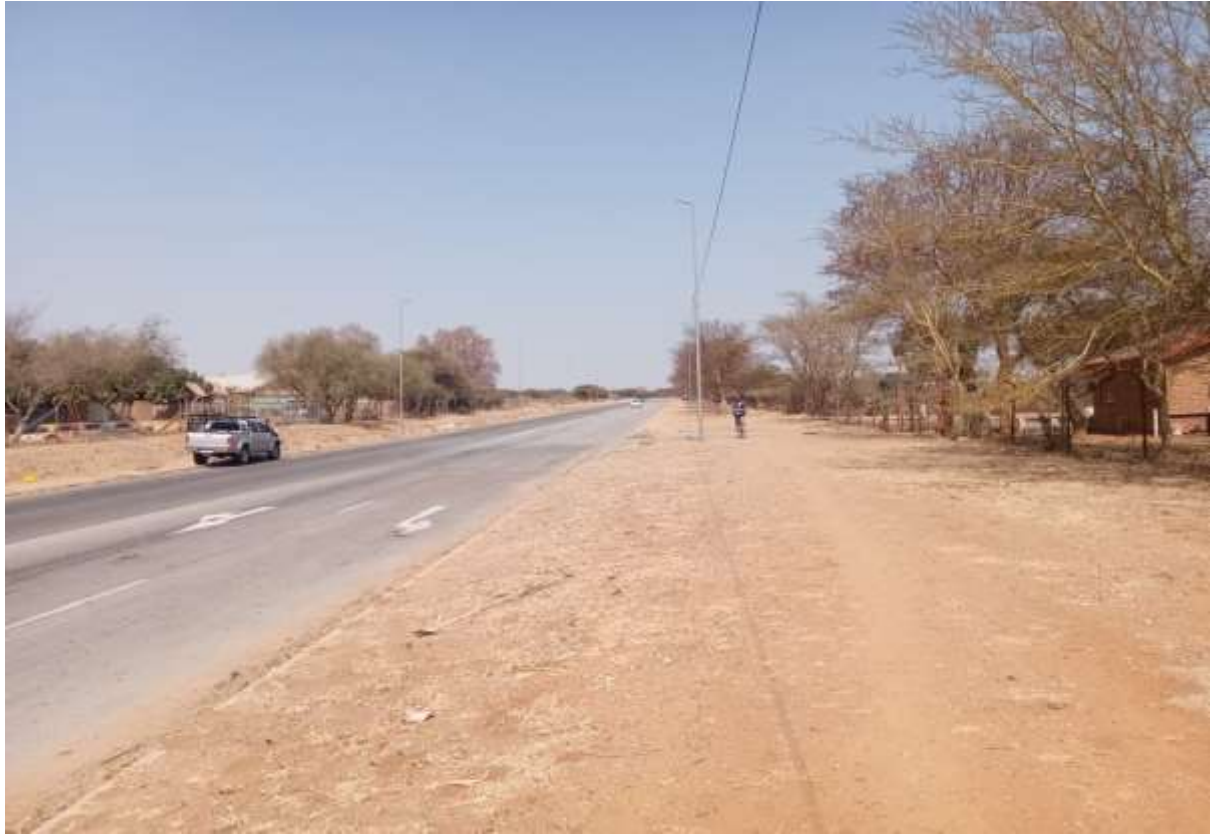
Figure 6: View of a road reserve portion where the proposed pipeline will run along Webster Street.
