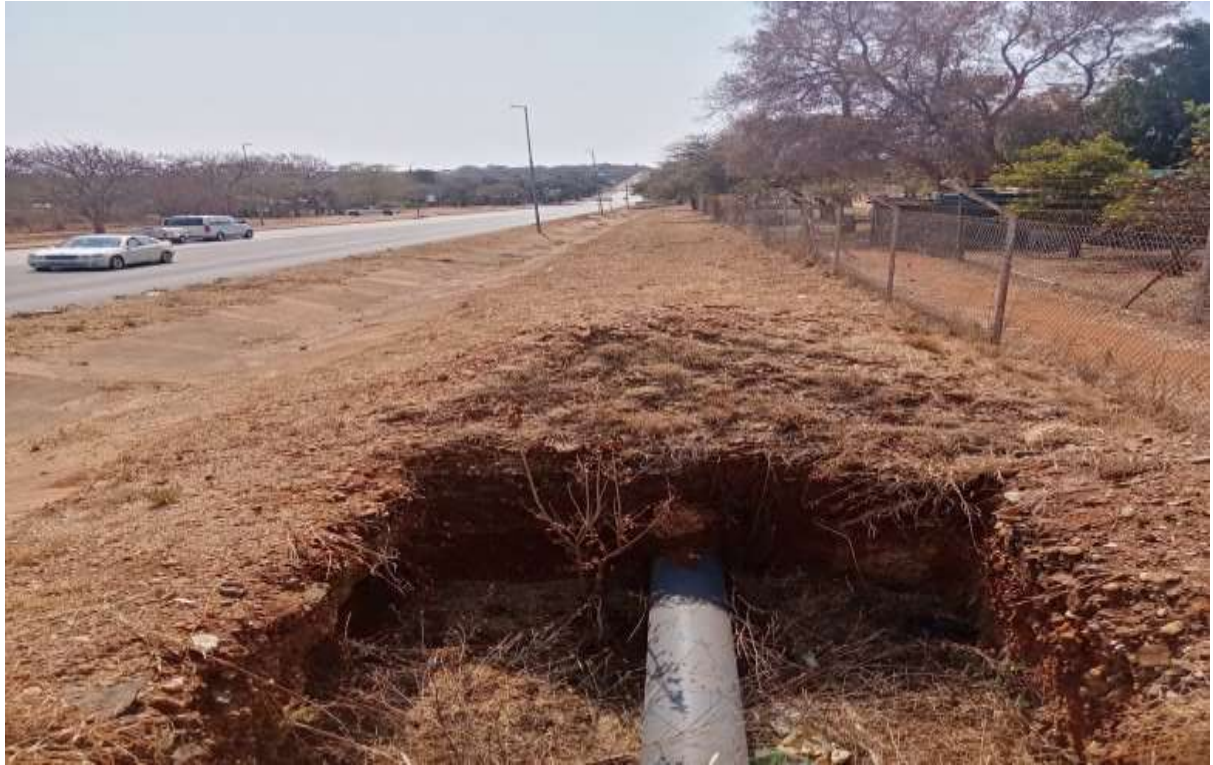
Figure 8: View of an existing pipeline along the road reserve. Note that the proposed pipeline will be laid much closer to the road before this existing pipeline
