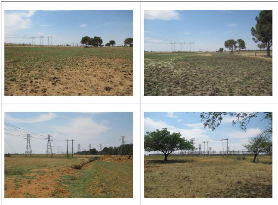
Figure 44: Views of the Phase 1 Power Line route (van Schalkwyk, 2020)
