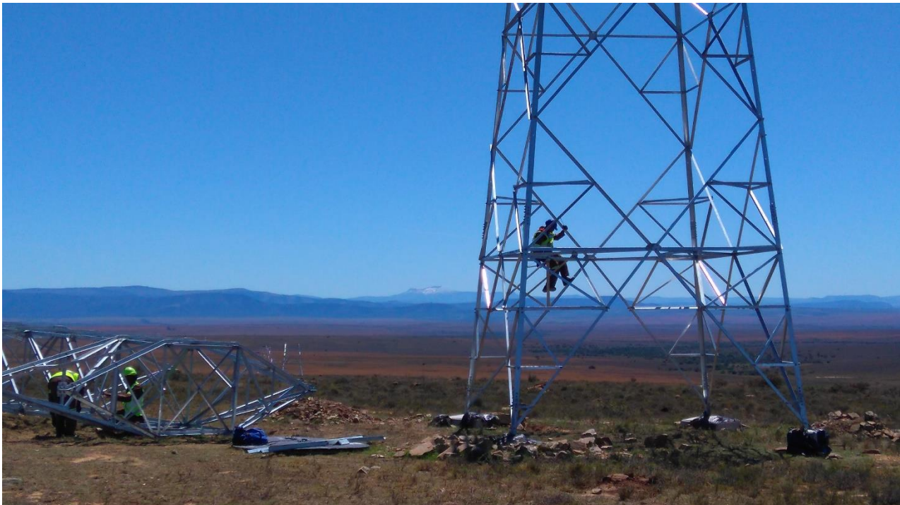
Figure 11: Example of a tower construction
