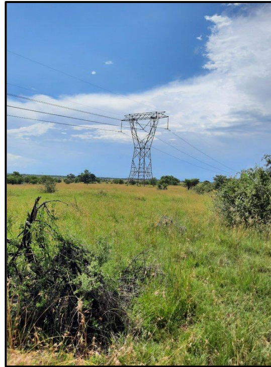
Figure 7.2. Existing powerlines traversing the study area.
