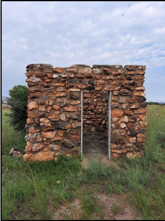
Figure 2.3. Rectangular structure at SF010.
