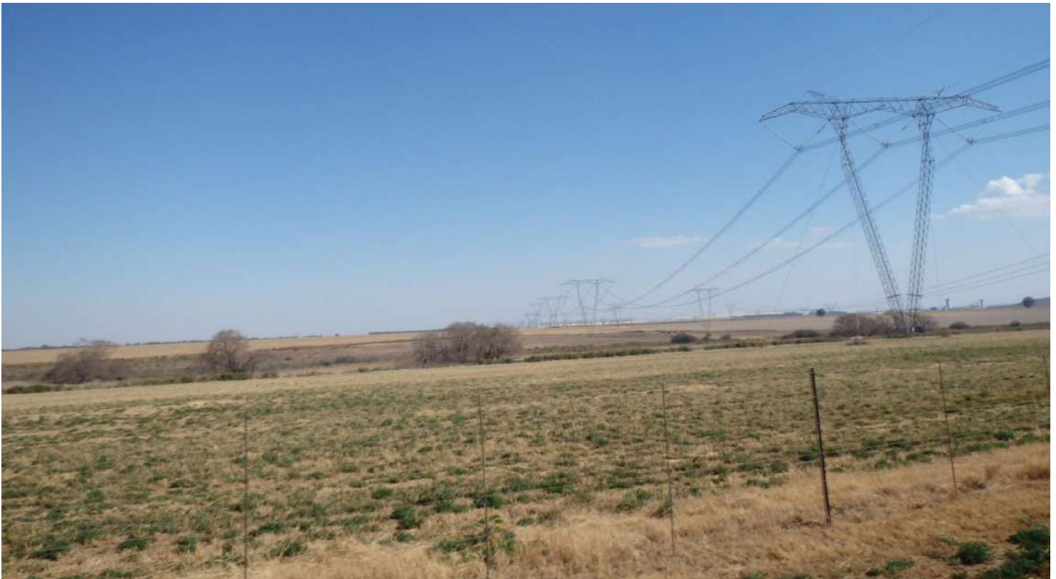
Figure 4.1: View of the existing OHL.
