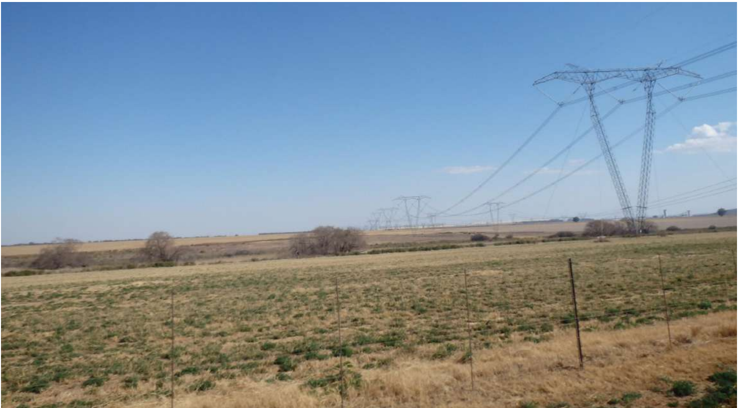
Figure 4.1: View of the existing OHL.
