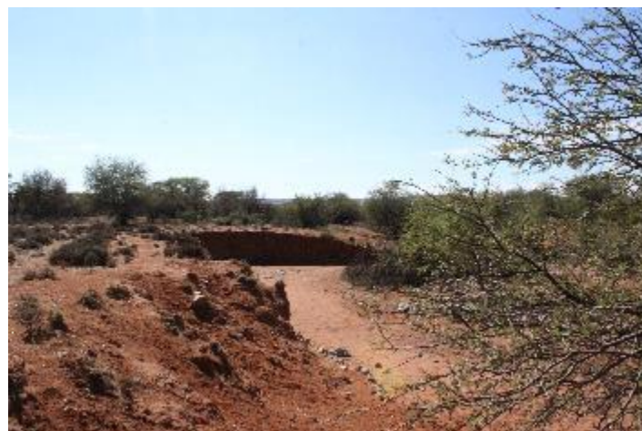
Figure 14: Several dry riverbeds and draining lines were observed throughout the project area.
