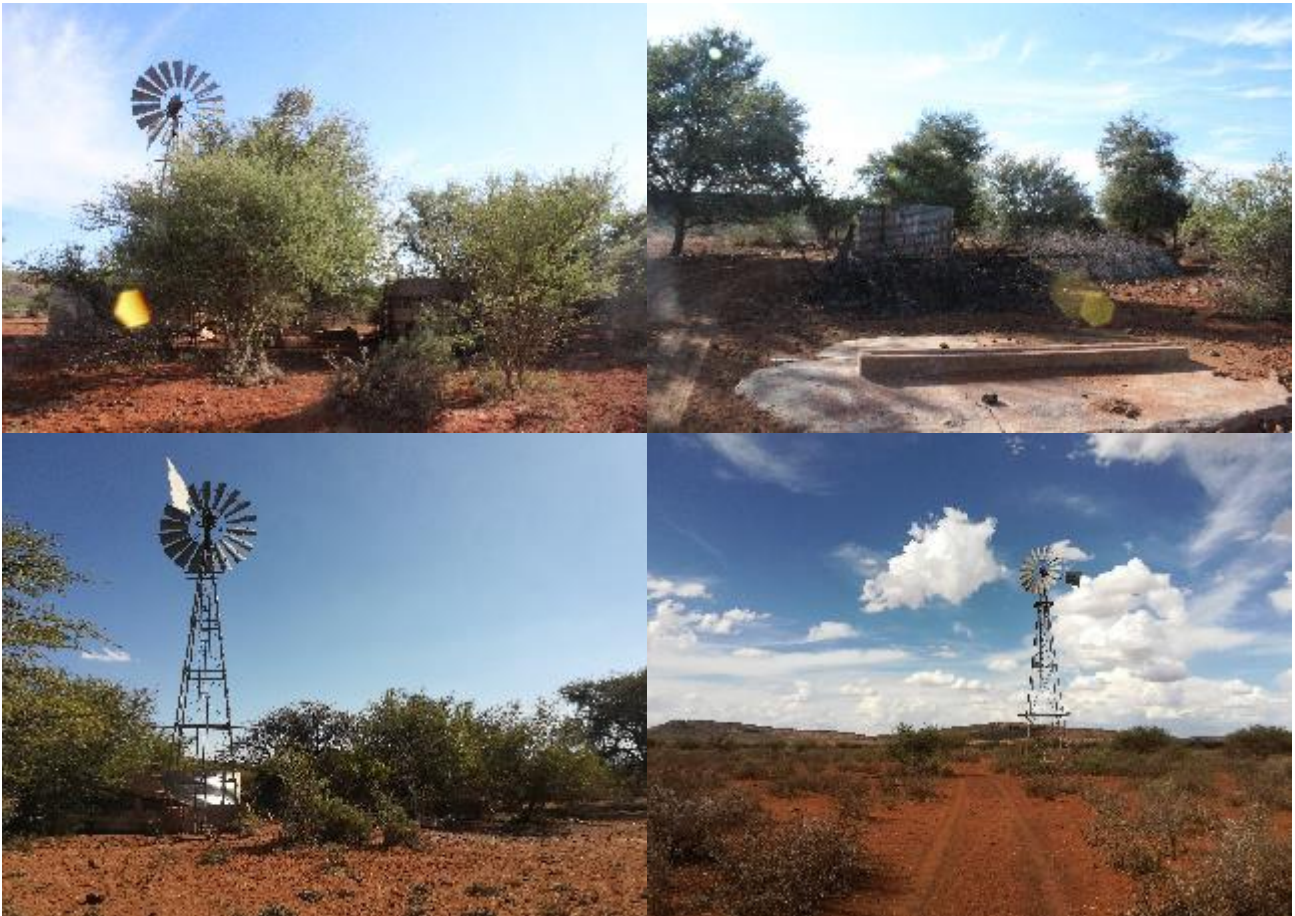
Figure 26: Wind pumps observed throughout the project area.
