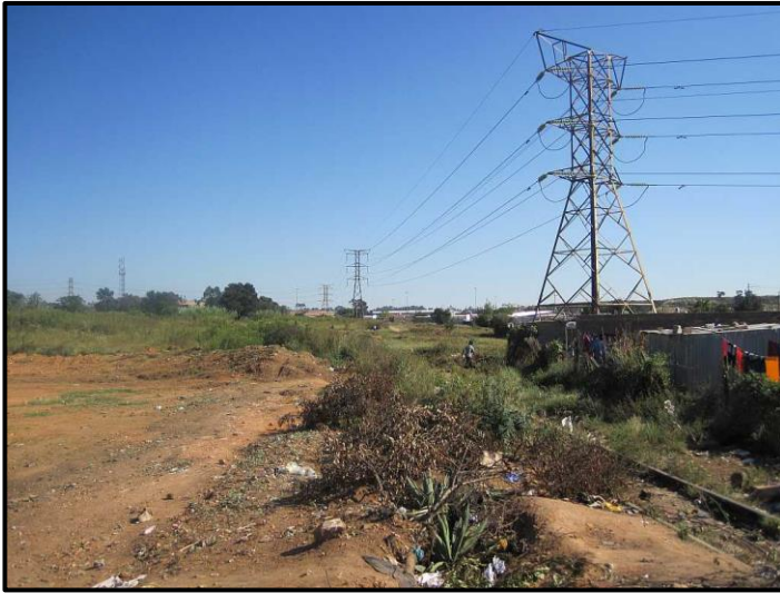
Figure 14. General site conditions – power line
