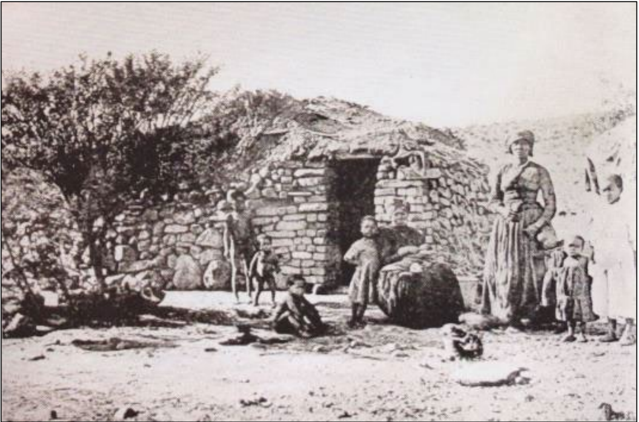
Figure 14: A shepherd's hut photographed near Beaufort West in the early 20th century. Note the low, narrow doorway and informal roof structure. Source: Schoeman (2013:48).
