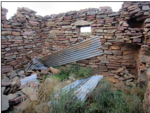
Figure 19: The interior of the north-eastern room in the ruin at waypoint 1980.
