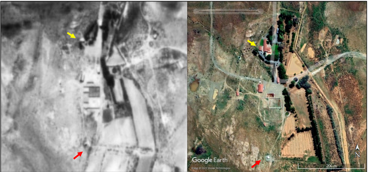
Figure 40: Historical aerial views from 1960 (434_005_02986) and today (Google Earth) of the Ystervarkspoort farmstead. Arrows show the corbeled building (red) and small outbuilding (yellow) behind the current farmhouse which does not seem to have been present in 1960.
