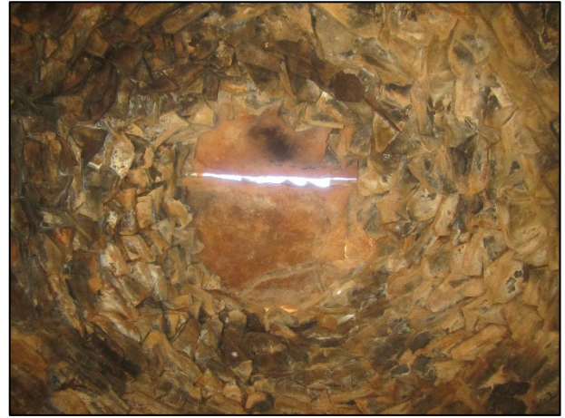
Figure 26: The inside of the dome in the corbelled building at waypoint 1270 showing two large slabs closing the top.
