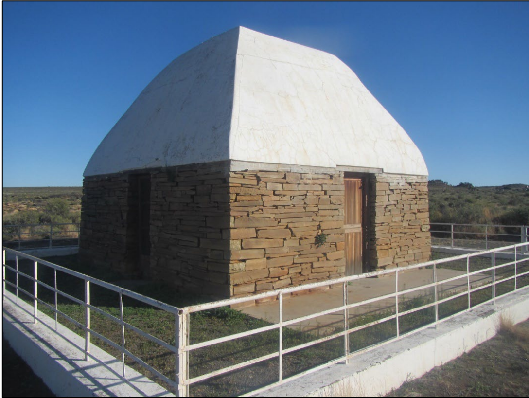
Figure 38: The corbelled building at waypoint 1265 and recorded as Ystervarkspoort 1 by Kramer (2012).
