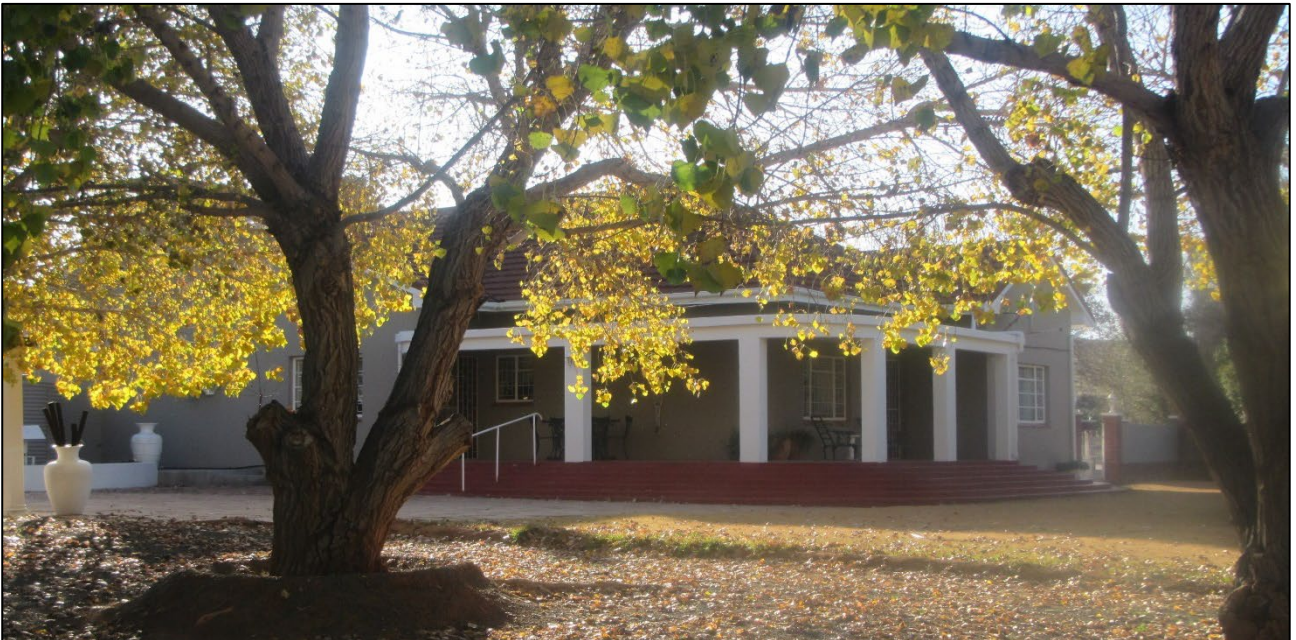
Figure 39: The current main farmhouse at the Ystervarkspoort farm complex at waypoint 1264.
