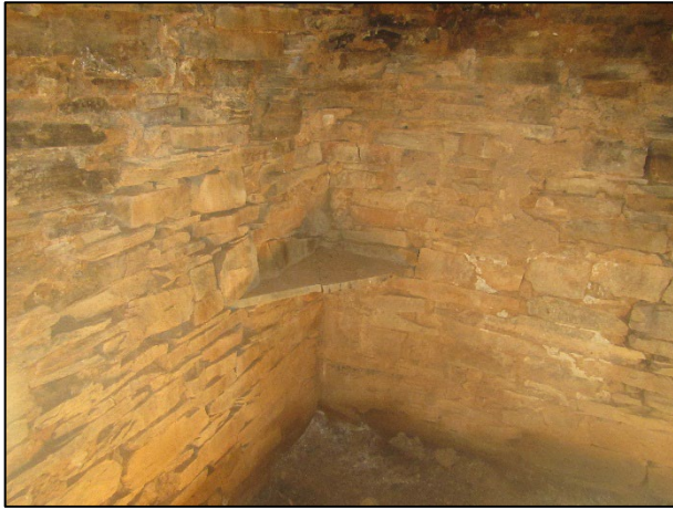
Figure 25: Internal corner shelf in the corbelled building at waypoint 1270.
