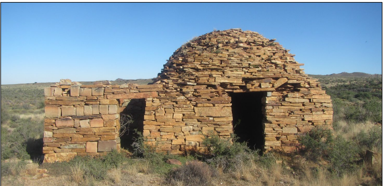
Figure 21: East and north sides of the corbelled building at waypoint 1270.
