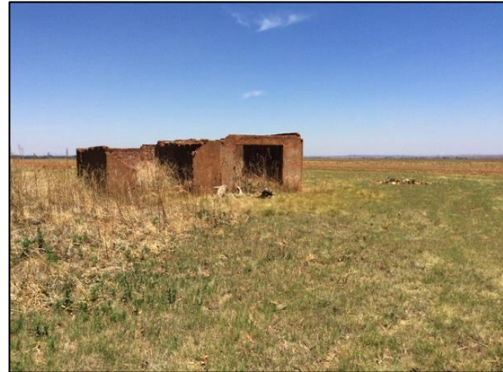
Figure 16 – View of the garage and store room at SB2
