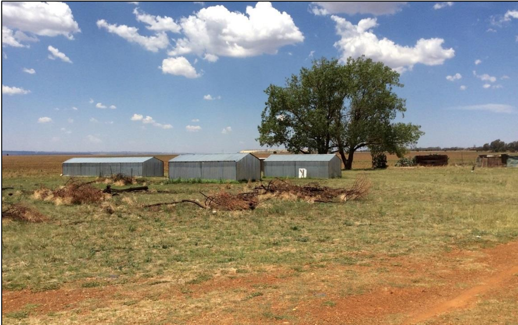
Figure 29 - New prefabricated houses at SB9
