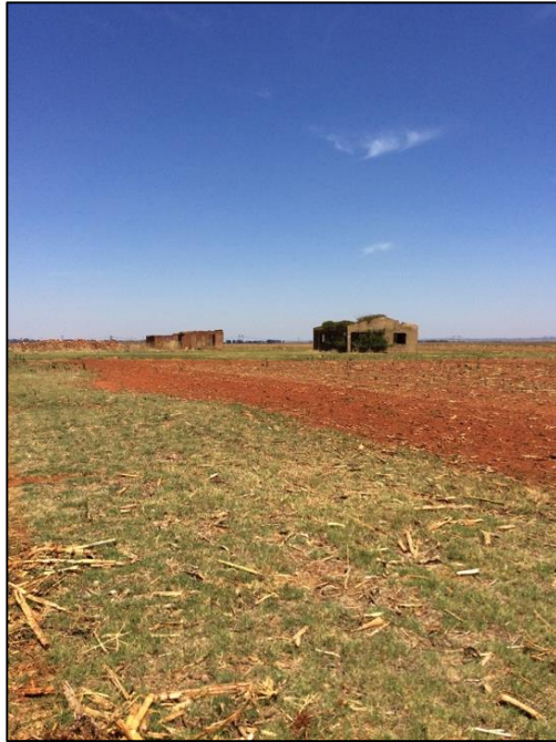
Figure 15 - View of SB2 from east
