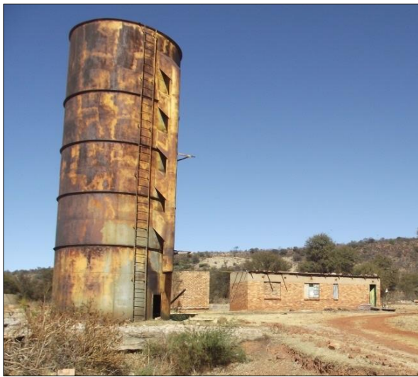
Figure 35 – Old silo & associated building
