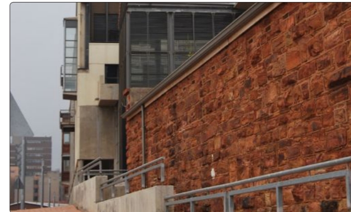
NORTH FACE OF STONE WALL TO NUMBER 4 AND 5
