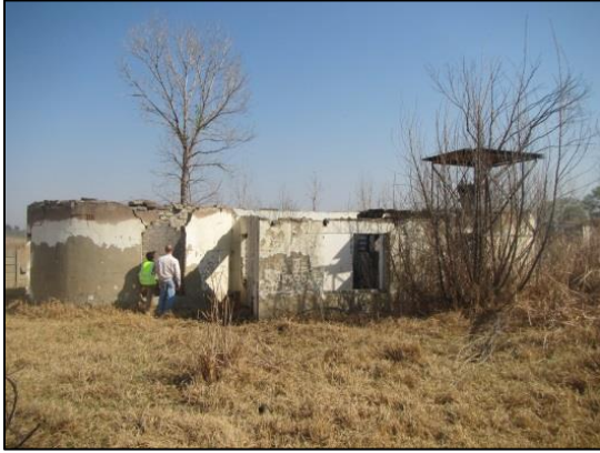
Figure 15- General view of the structure at Sas2
