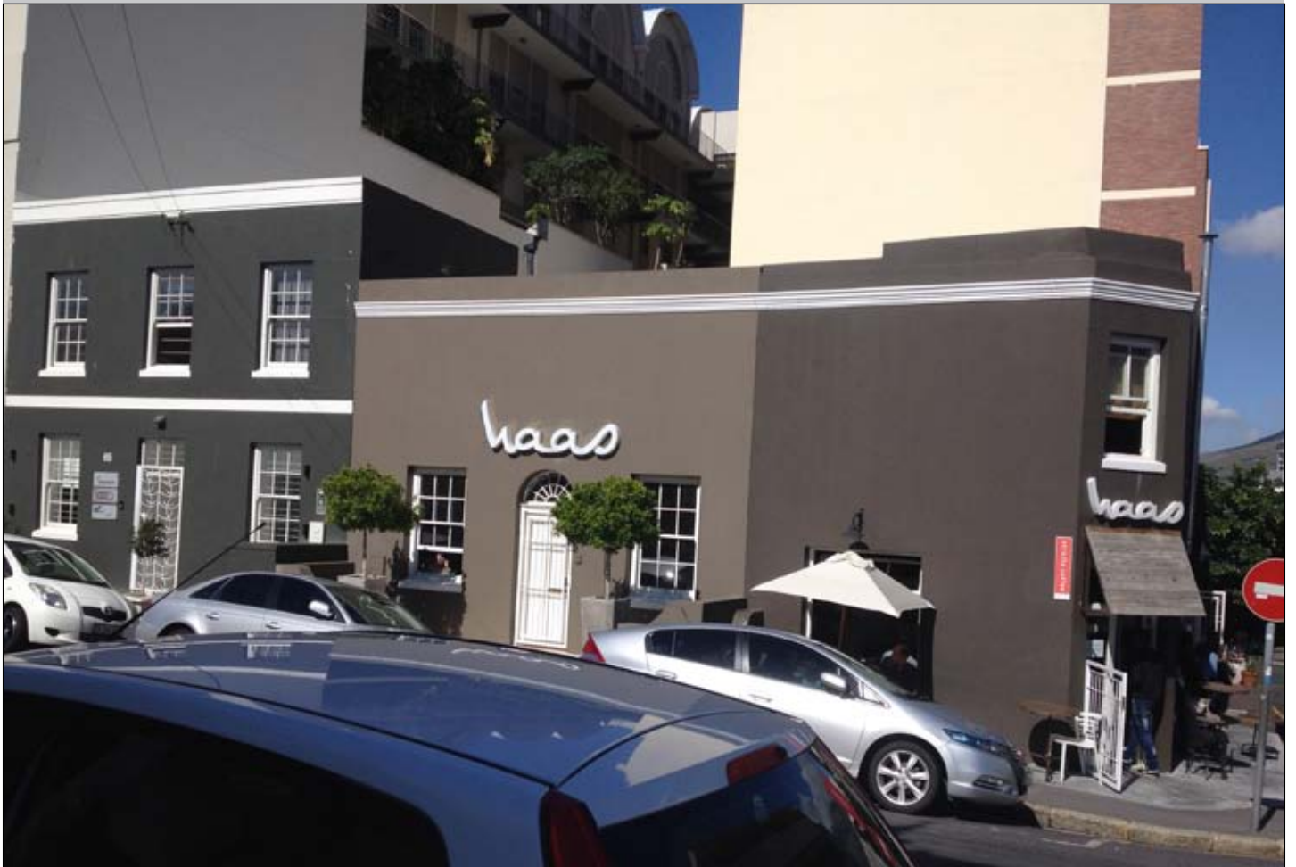
Figure 23: Three adjoining row houses, typical of the historic core of Bo Kaap, have been well maintained outside of the wider Provincial Heritage Site/Area. All three enjoy MU3 Zoning.
