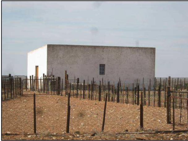
Figure 18: A mid-20 th century outbuilding at KOE2012/005.
