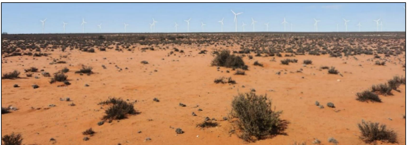
Figure 5: View across the proposed BESS area (note that the substation has yet to be built. The turbines in view are the adjacent Kangnas WEF). Source: Liandra Scott-Shaw (SiVest).
