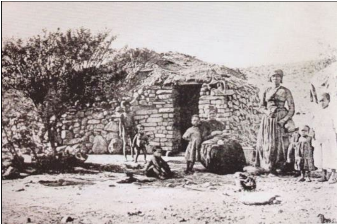
Figure 14: A shepherd's hut photographed near Beaufort West in the early 20th century. Note the low, narrow doorway and informal roof structure. Source: Schoeman (2013:48).
