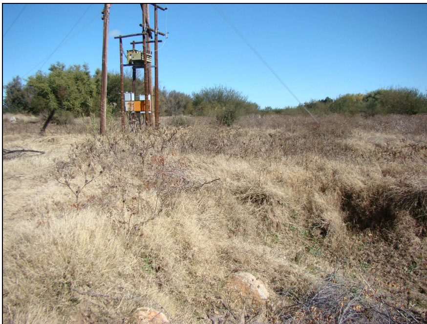
Fig.1 Point C at Melkstroom 563, Upington.
