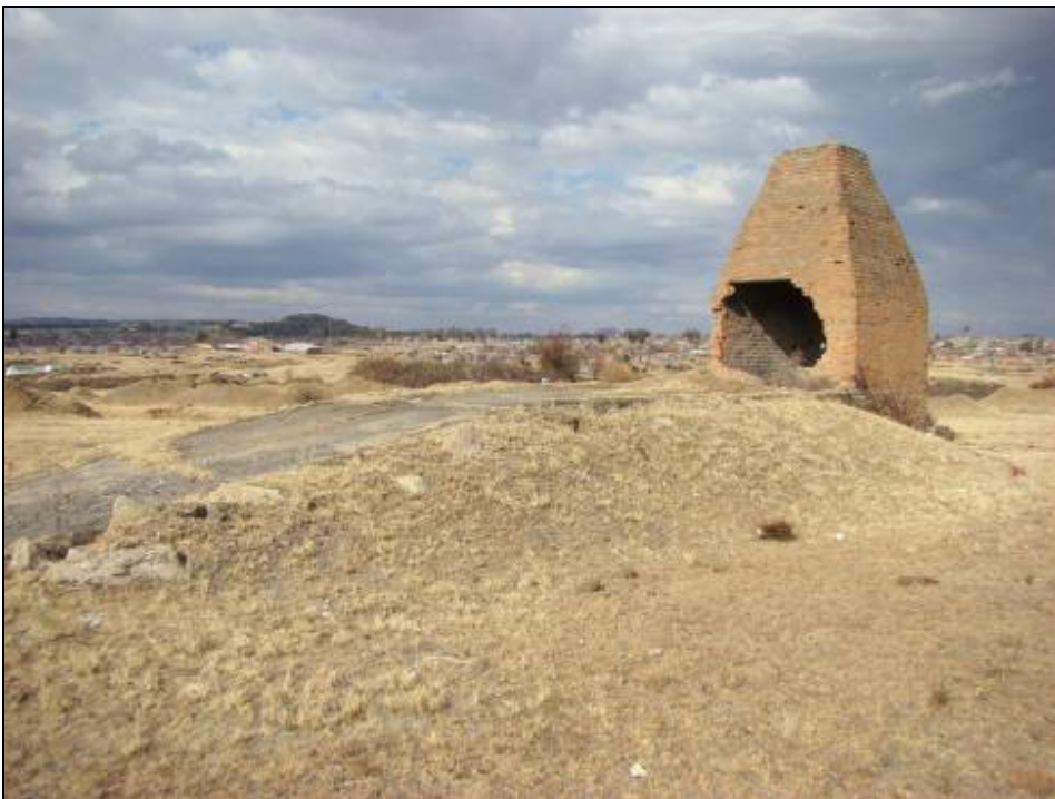
Fig.11 The old incinerator at the dumping site at Clocolan.
