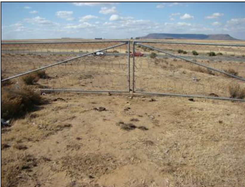
Fig.15 Entrance gate between Point A & C at the solid waste site Senekal.
