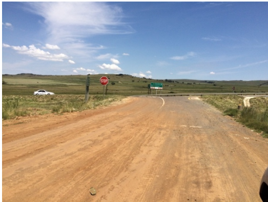
Figure 2 –Junction of D281 and N11 (southern end of D281)
