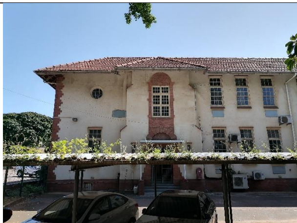
View of building from east.
