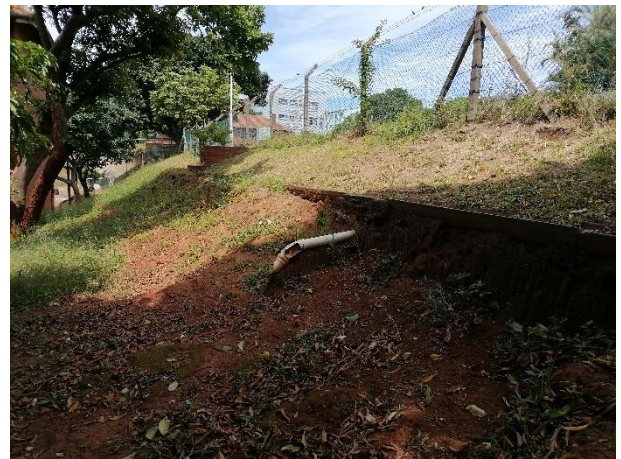
Open channel drain.
