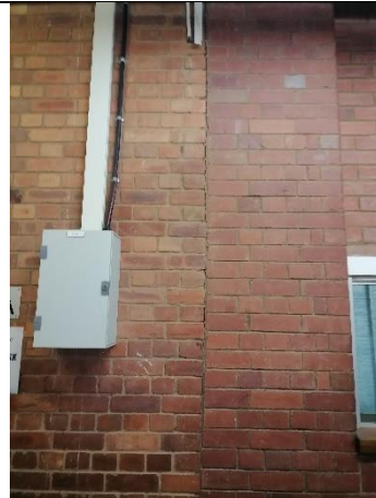
Construction Joint.
