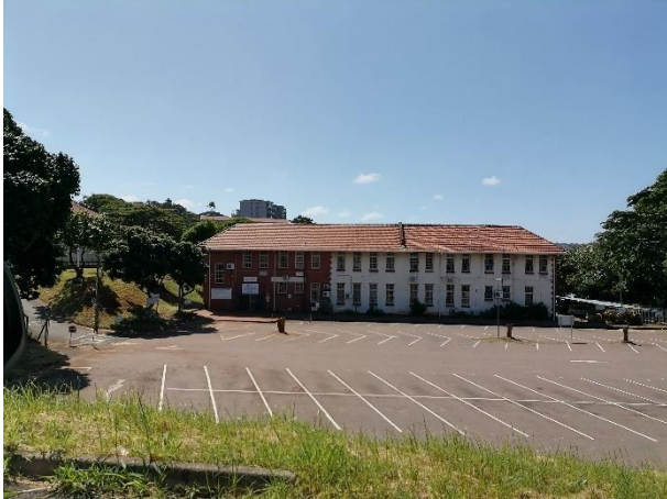
Front view of building.
