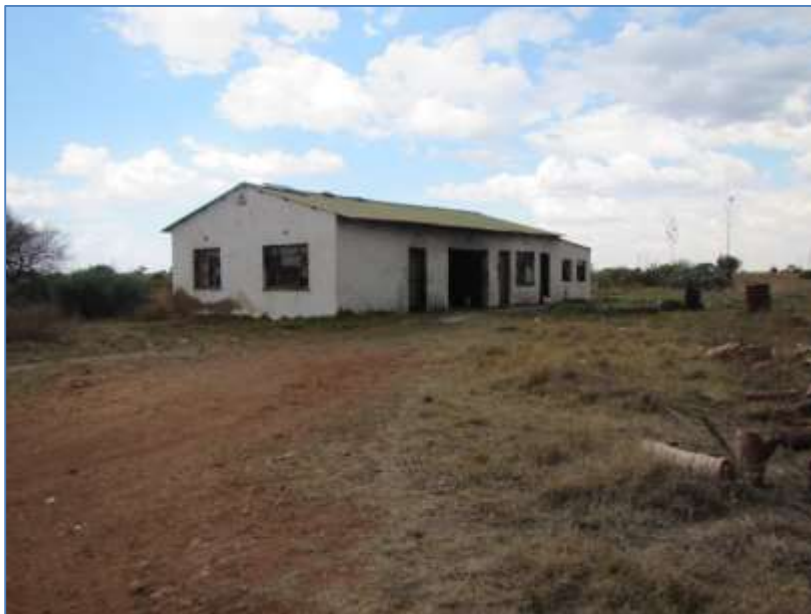
Figure 7 – derelict farmhouse at TS02
