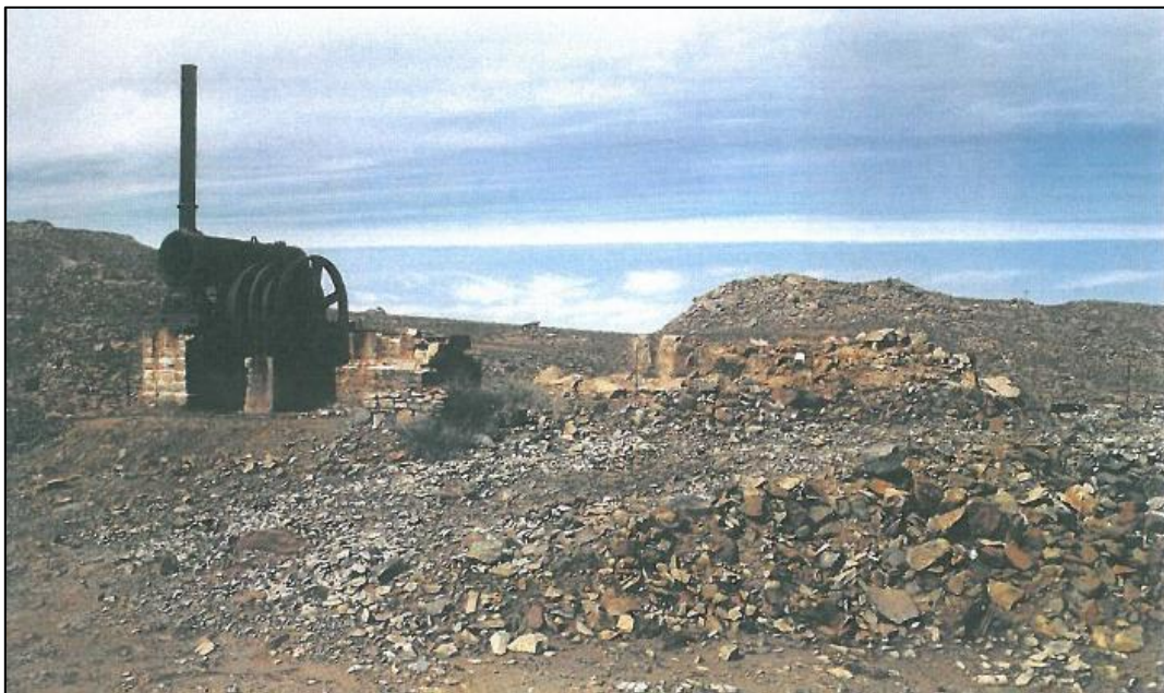
Figure 28: The Narap Mine with the remains of an old steam engine as seen in 1993. Source: Cairncross (2004:303).
