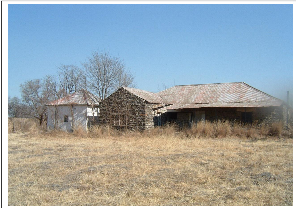
Figure 5- A residence with outbuilding on Vaalbank 358. The house was built with dolerite and is fitted with a pitched corrugated iron roof. Together with a clay dwelling these structures constitute FC02 (above).
