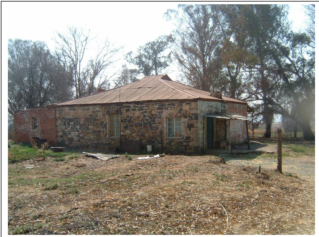
Figure 13- HH04 on Khadie 1309 was constructed with dolerite. The house was renovated and is currently fitted with steel window frames while a lean-to which was constructed with clay bricks was added to the house's back side (above).
