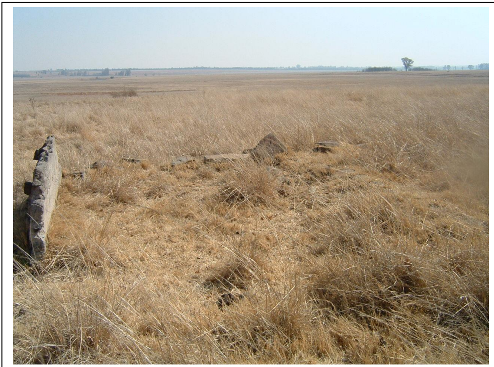
Figure 4- Foundations of a one-roomed structure which was constructed with dolerite. The cement wall probably replaced an original mud wall (above).
