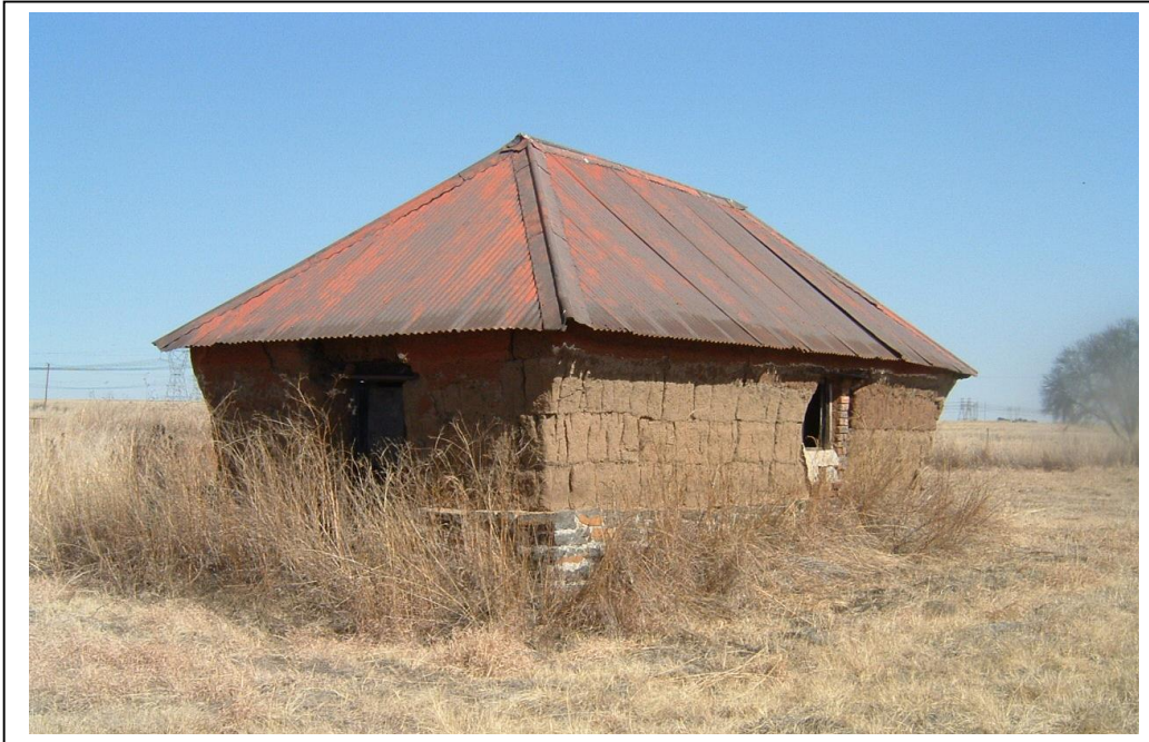
Figure 6- A dwelling with dolerite foundations and clay walls in FC02. Note the clay sods (bricks) with which the walls were constructed. This may be one of the oldest buildings in the NVC Project Area (above).
