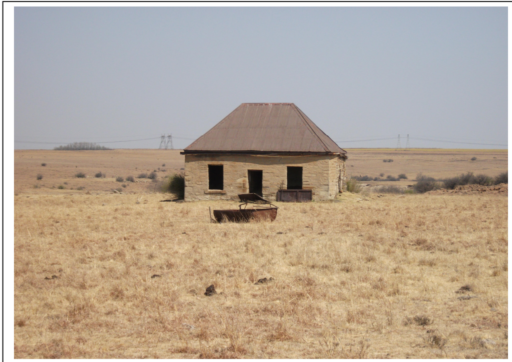
Figure 9- A sandstone dwelling with pitched corrugated iron roof is part of FC06. It seems as if this structure was constructed with building material which once was part of a British blockhouse (above).
