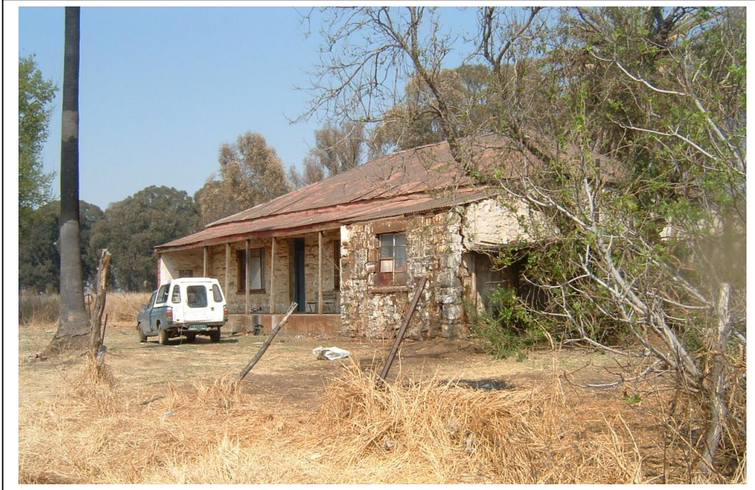
Figure 11 - The main residence in FC08 was constructed with dolerite. It is associated with a wagon shed and a rondavel which has been turned into a silo (above).
