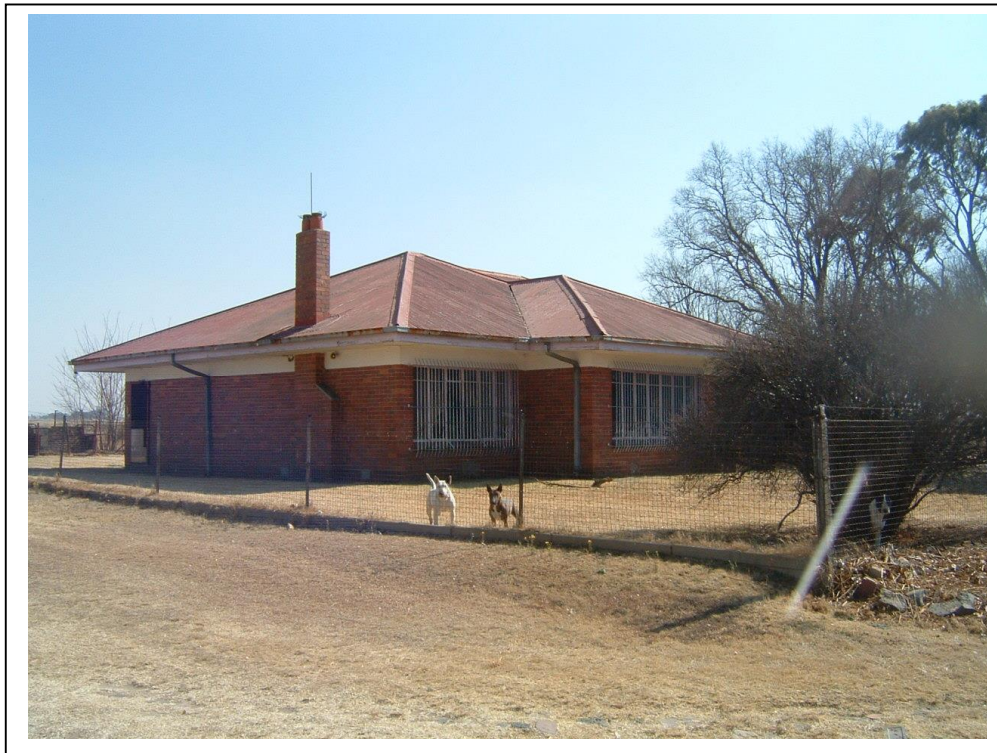
Figure 12- Historical House 03 on Vaalbank 238 was constructed with red face clay bricks and with cement and probably dates from the 1950's or 1960's (above).
