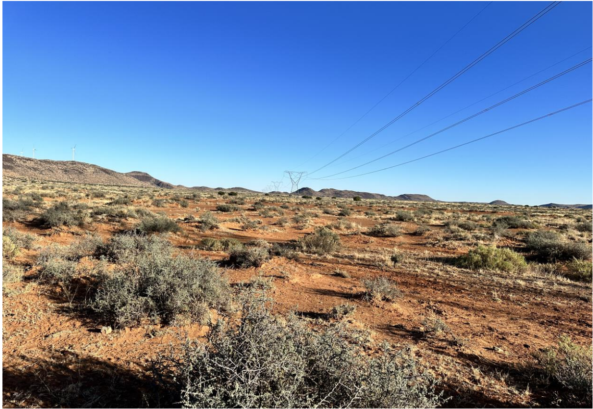
Figure 2: General site overview of the area proposed for construction from Kronos substation.
