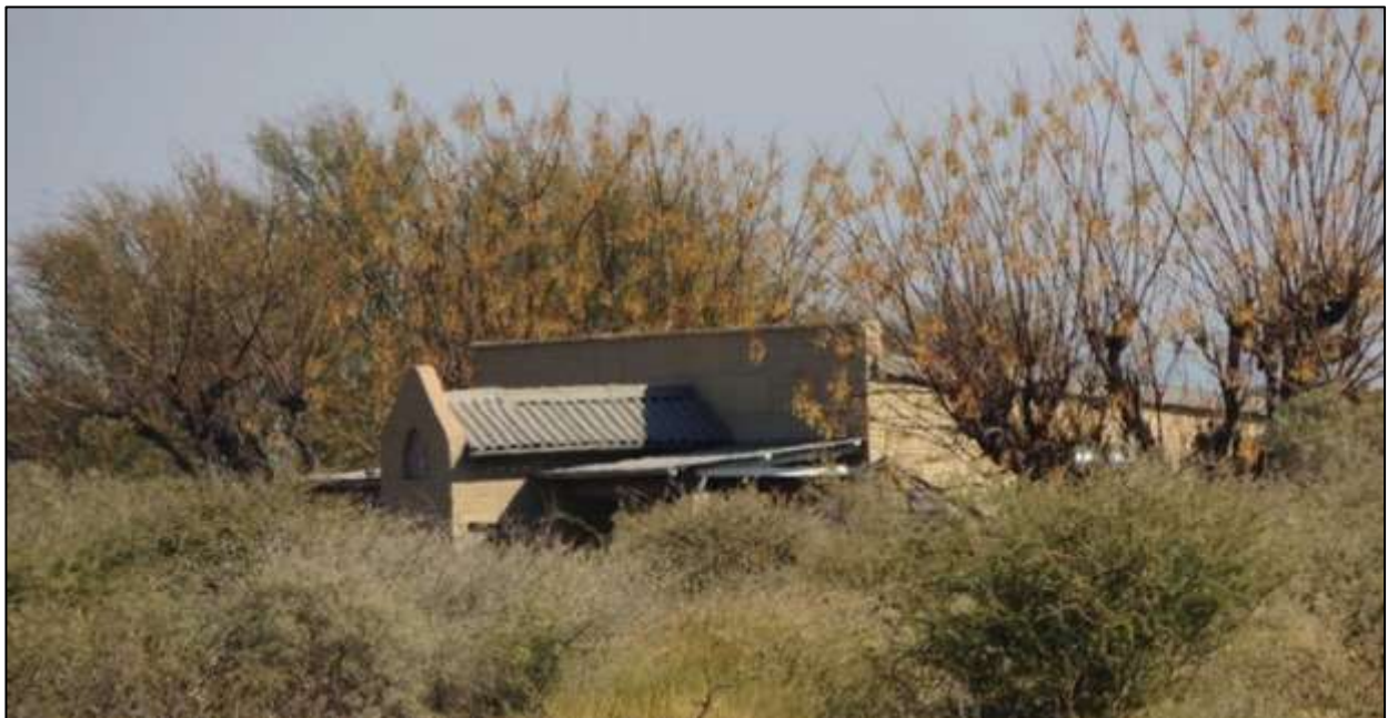
Figure 16: Photograph of an isolated farmhouse, which is located on the proposed property, as seen from the R31.
